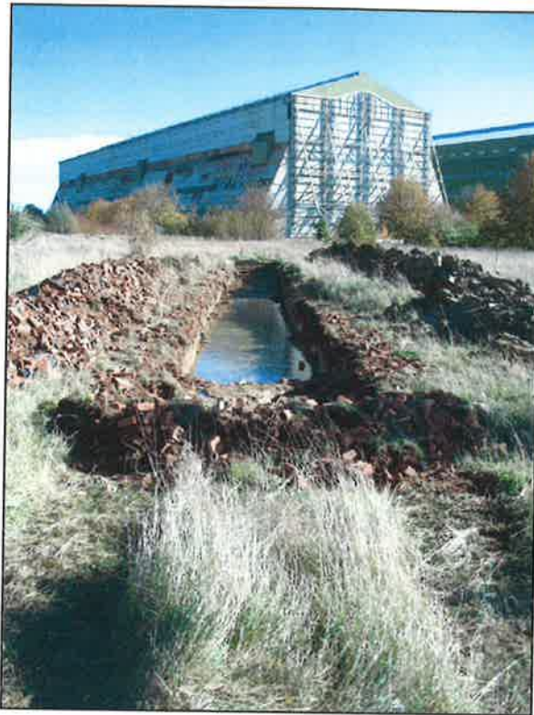
Plate 1 Trench 3 and hangars
