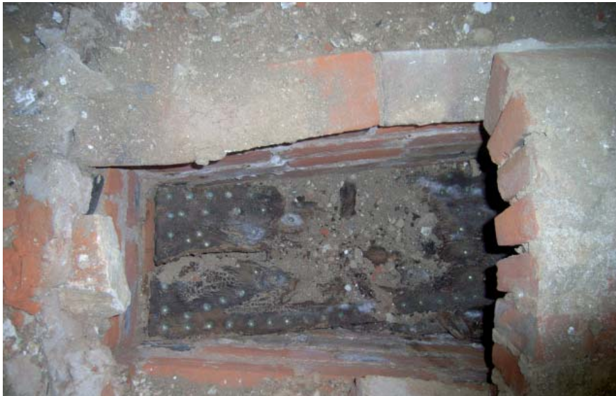
Plate 13: Brick vault (2003) truncating E-W section of original north wall (2007)
