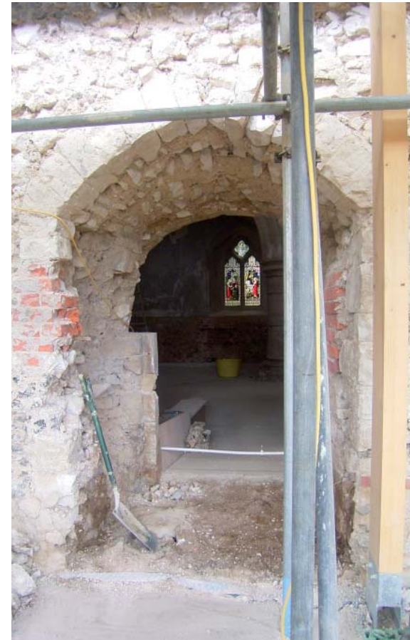
Plate 26.: South elevation showing Nun's doorway after unblocking
