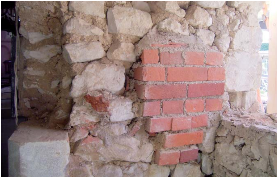
Plate 25: West wall of Nun's doorway passage showing red brick repair
