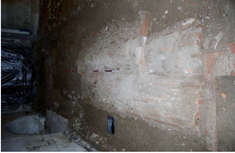
Plate 15: Brick lined vaults revealed within north wall
