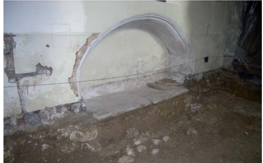
Plate 12: Above ground niche; eastern end of north wall of north aisle
