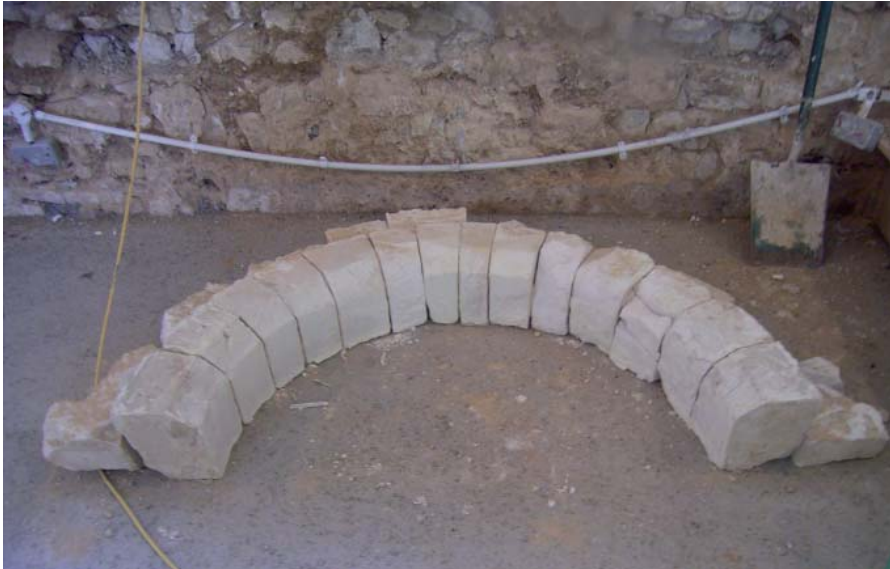
Plate 24: Interior arch from Nun's doorway having been removed
