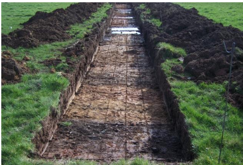
Plate 5: South facing view of Trench 4
