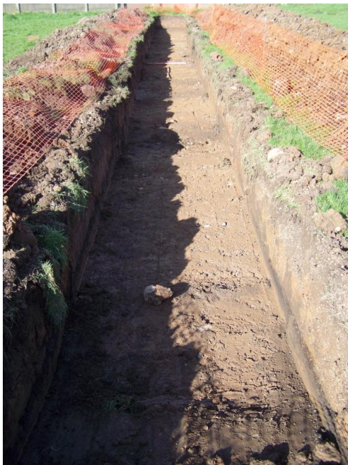
Plate 1: North facing shot of Trench 1
