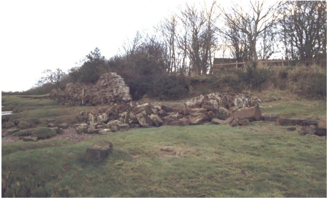
Plate 7: Site 83 , ruined sea defences, looking south-east
