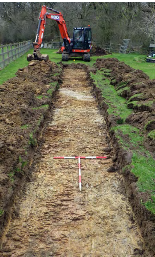
Plate 3: Trench 7, view to north
