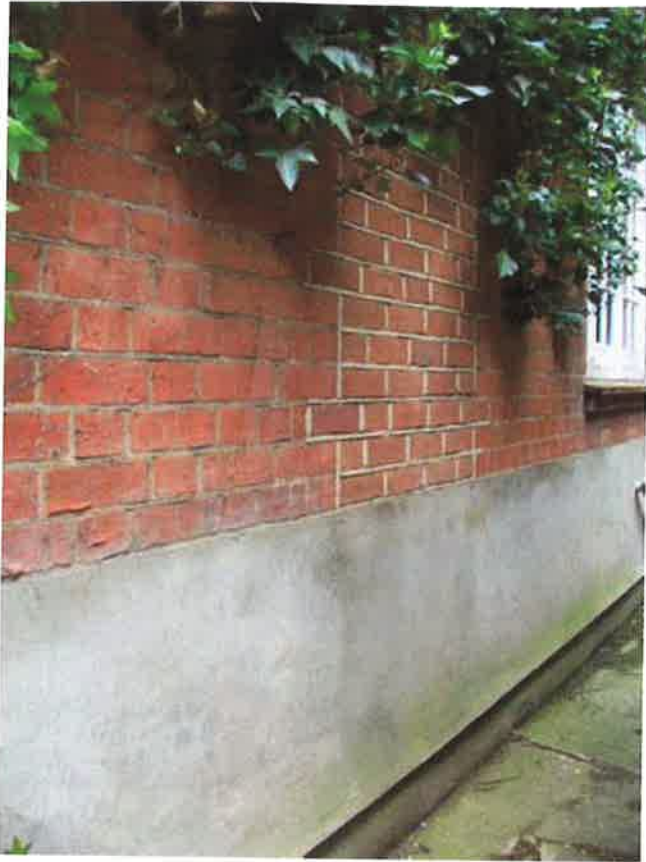
Plate 7: View of the east elevation facing northwest, showing the blocked up doorway
