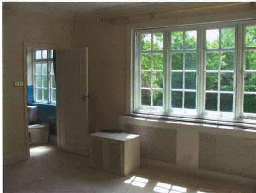
Plate 18: View of F8 looking southeast, showing doorway to F7
