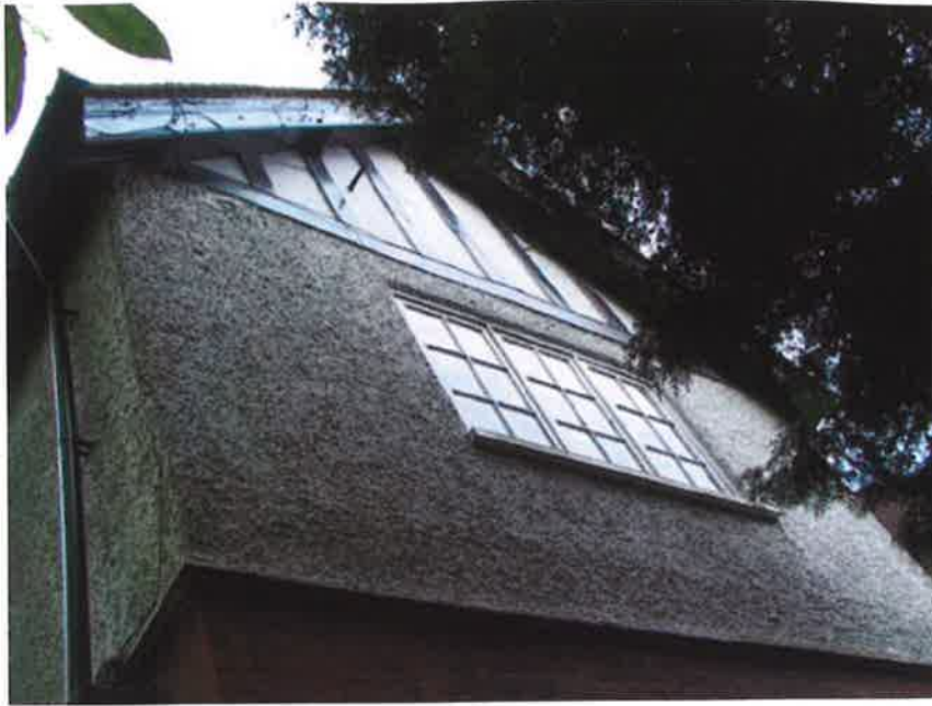
Plate 5: View of the magpie-work on the north elevation
