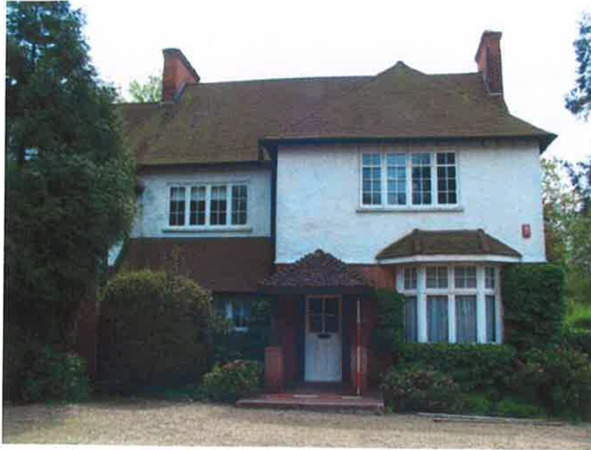
Plate 1: View of the front (north elevation) of the property, facing south
