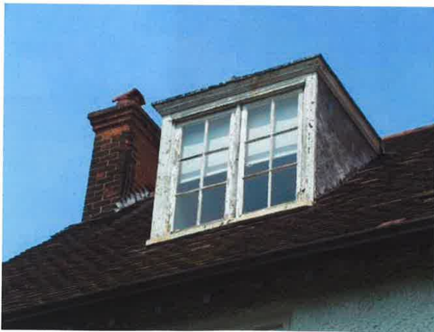
Plate 4: View of the western chimney and dormer, facing northwest
