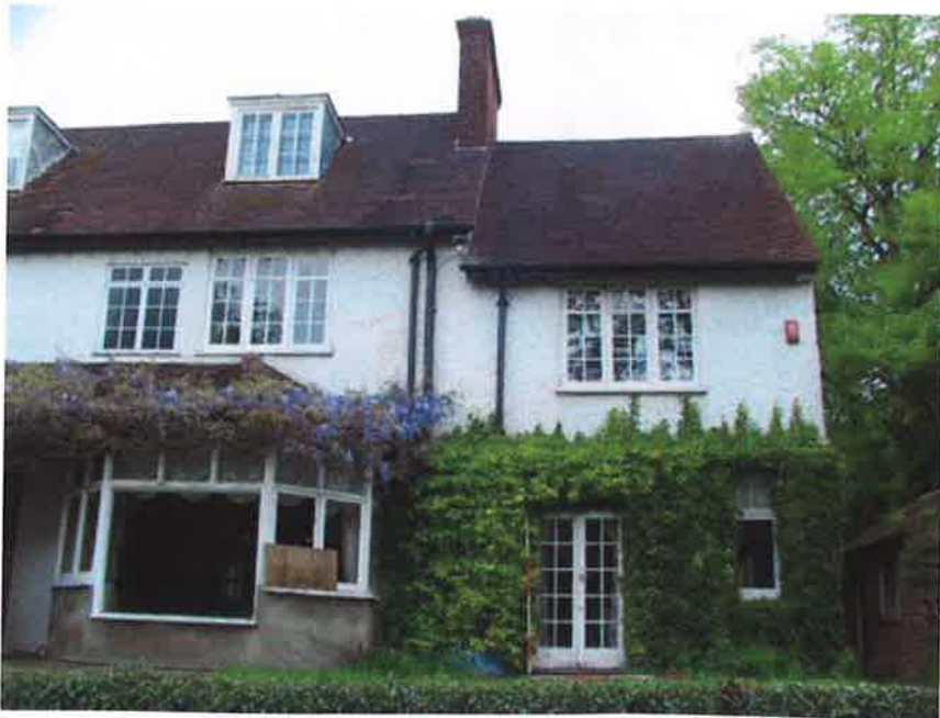
Plate 8: View of the eastern half of the south elevation, facing north
