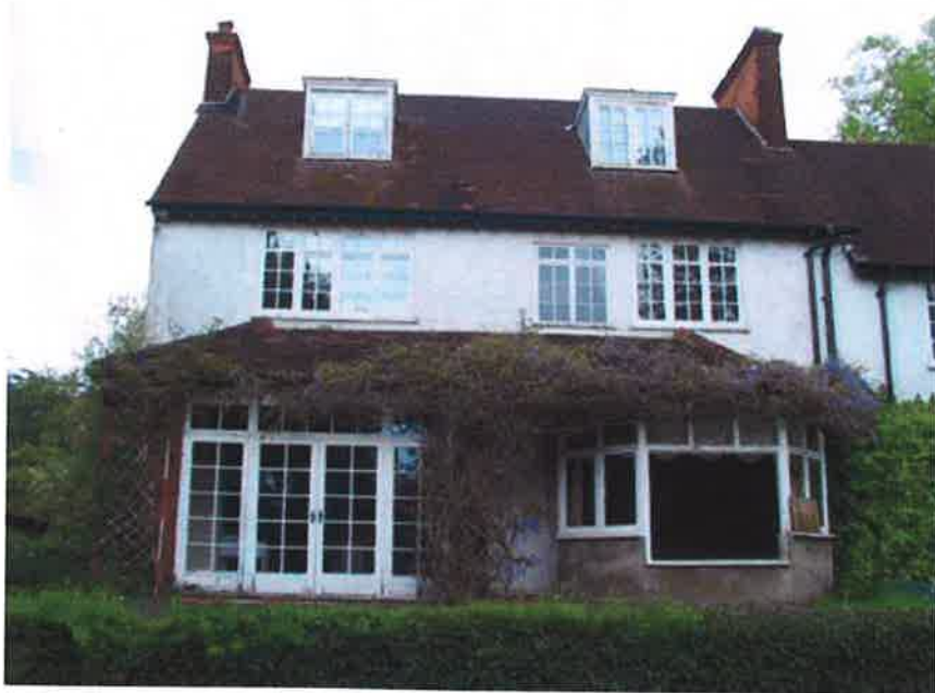
Plate 2: View of the rear (south elevation), facing north
