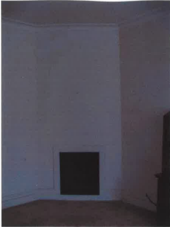
Plate 13: View of G2 facing southwest
