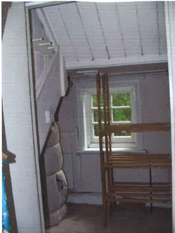
Plate 17: Linen cupboard (F3), used as an airing cupboard/hot water storage
