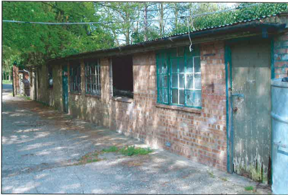
Plate 1: WW2 building, looking north
