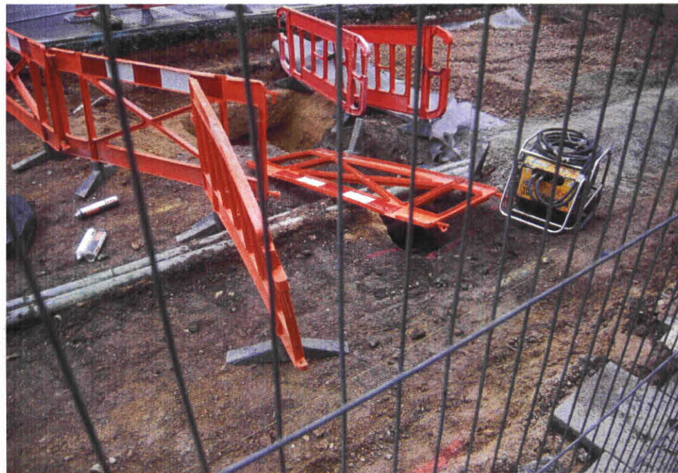
19) Service trench, section 3 → N
