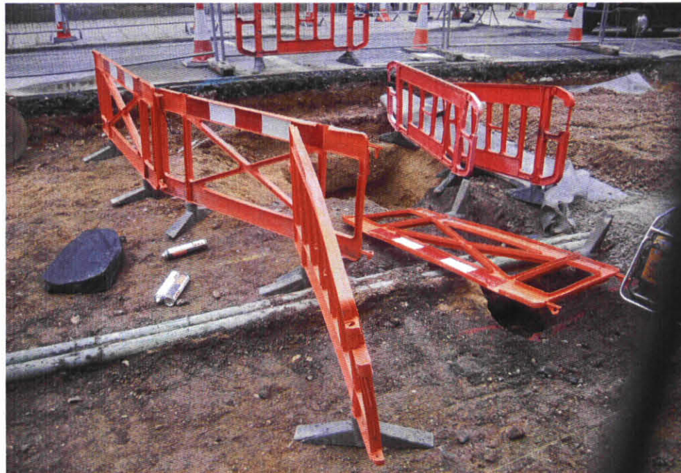
20) Service trench Section 3 → N
