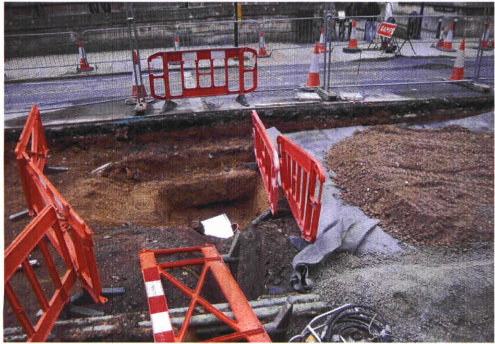
22) Service trench Section 3 → N
