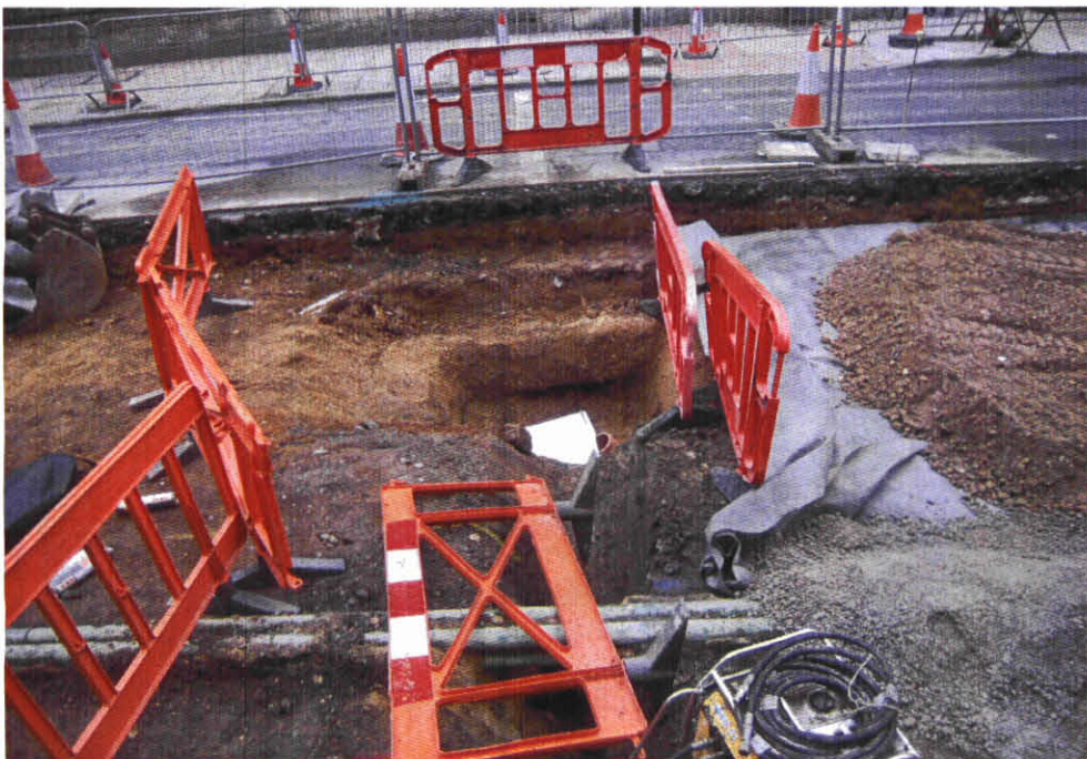
17) Service trench, section 3 → N
