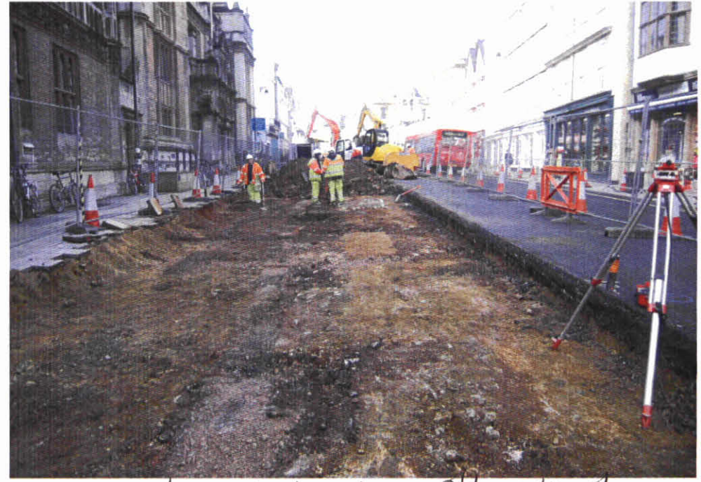
31) Reduction of level, south side of High St, Junction Merton St. → W
