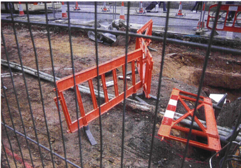
18) Service trench, section 3 → N
