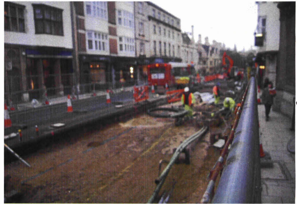
16) Excavation of N. side of High street → W
