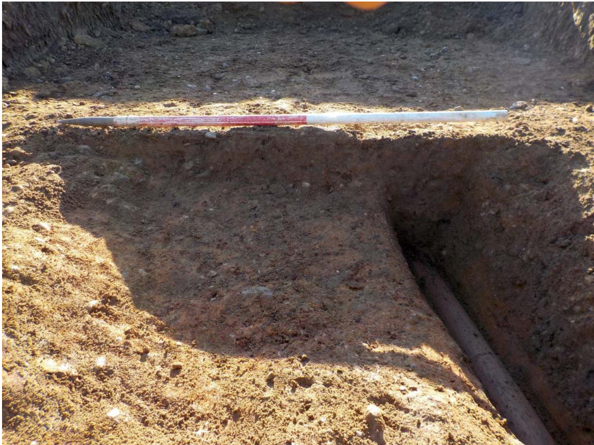
Plate 16: Ditch 7203 and drain 7205, looking south
