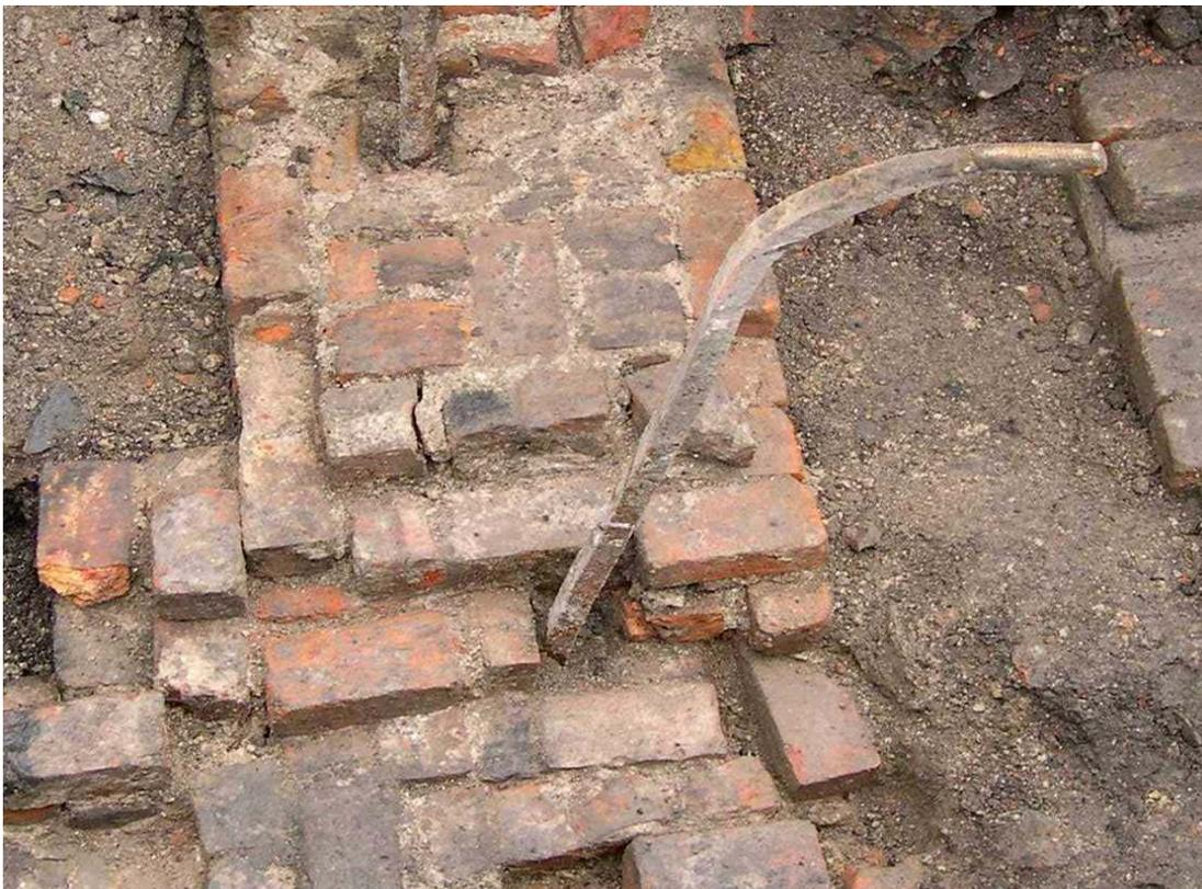
*Plate 3: Engine restraining rod within central part of foundation structure **05***
