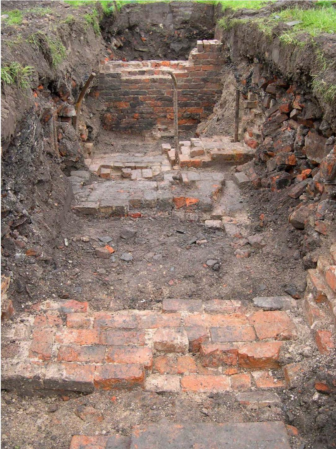
*Plate 1: Structural remains encountered within the south-eastern part of Trench 1. Wall **04** lies in the foreground and wall **06** to the rear, with the foundations (**05** and **11**) for a steam engine situated in between.*
