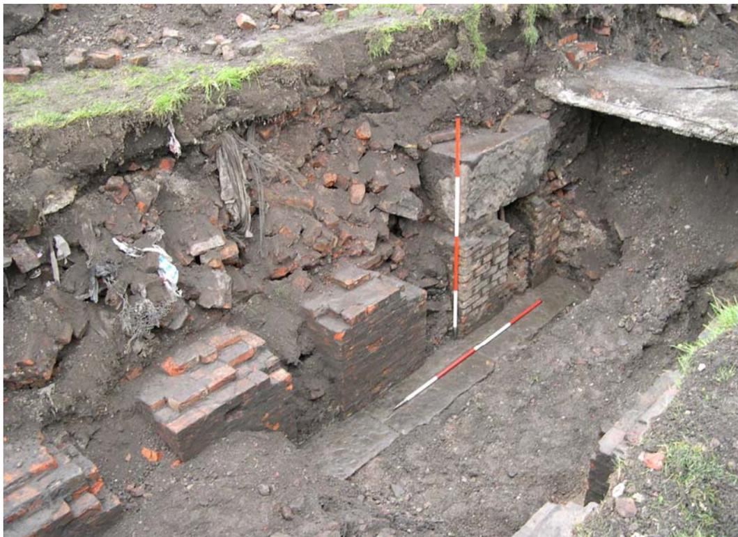
*Plate 7: Part of a series of brick piers encountered within Trench 2*
