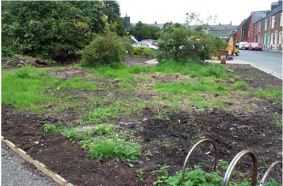
Plate 1: The site prior to work being carried out, looking north-west
