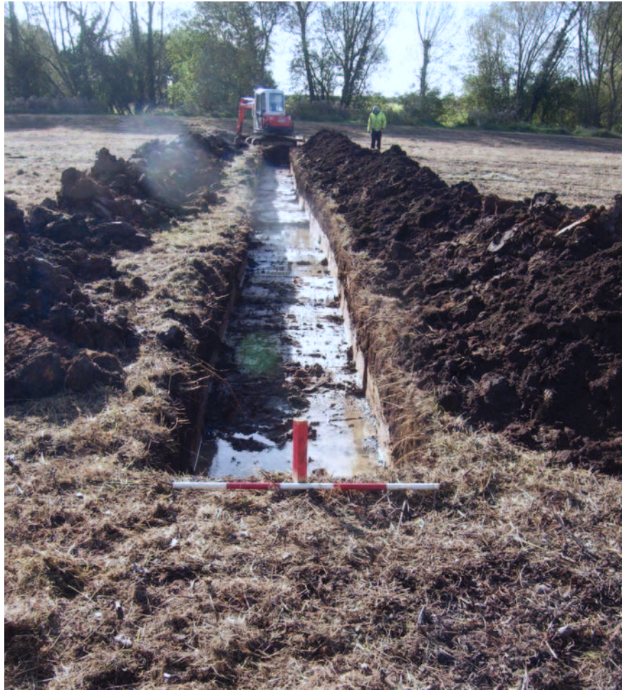
Plate 5: Photo of Trench 4 looking south
