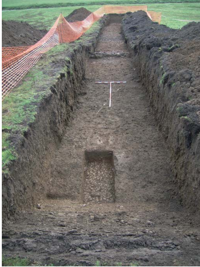
Plate 9: Trench 8 view to north-west
