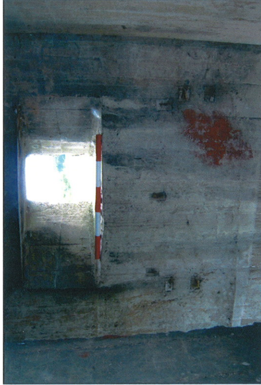
Plate 10: Interior view of south embrasure showing timber fixing blocks below, 0.5m scale
