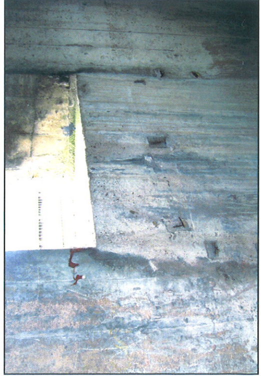
Plate 7: Interior showing west embrasure looking north-west
