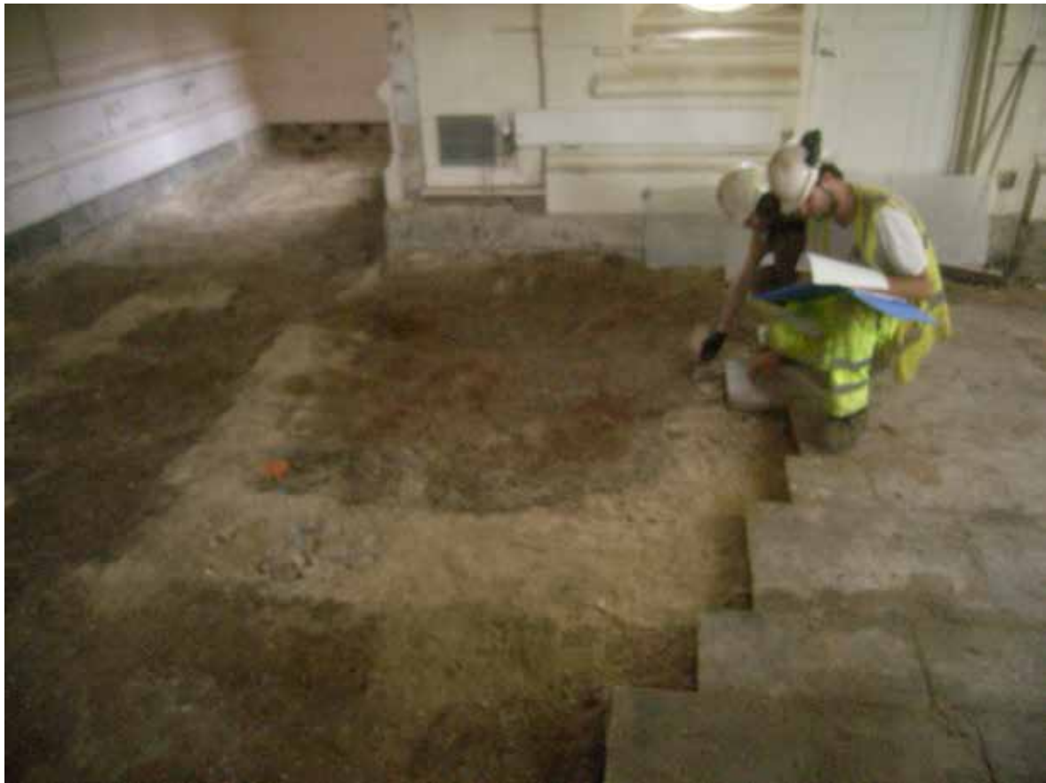
Figure 13: Cleaning back after removal of floor slabs
