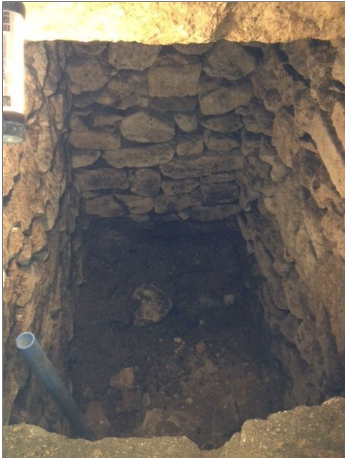
Figure 25: Stocker Room, Cistern
