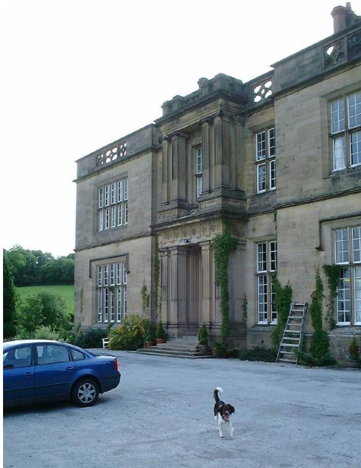
Plate 3: Front, East, External Elevation, South End, Looking South-west
