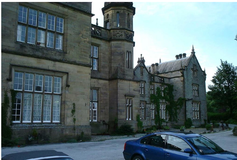
Plate 4: Front, East External Elevation, North End, Looking North-west
