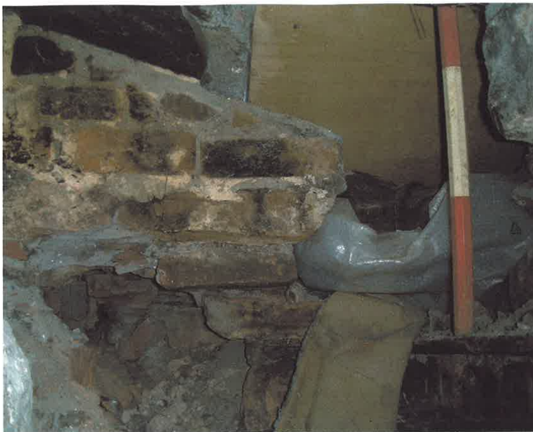
Plate 3: Detail of the brick and slate construction of the flue within 106
