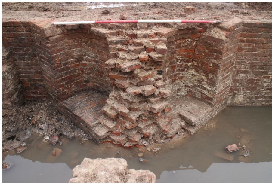
Plate 2: East-facing view of boiler stands 102
