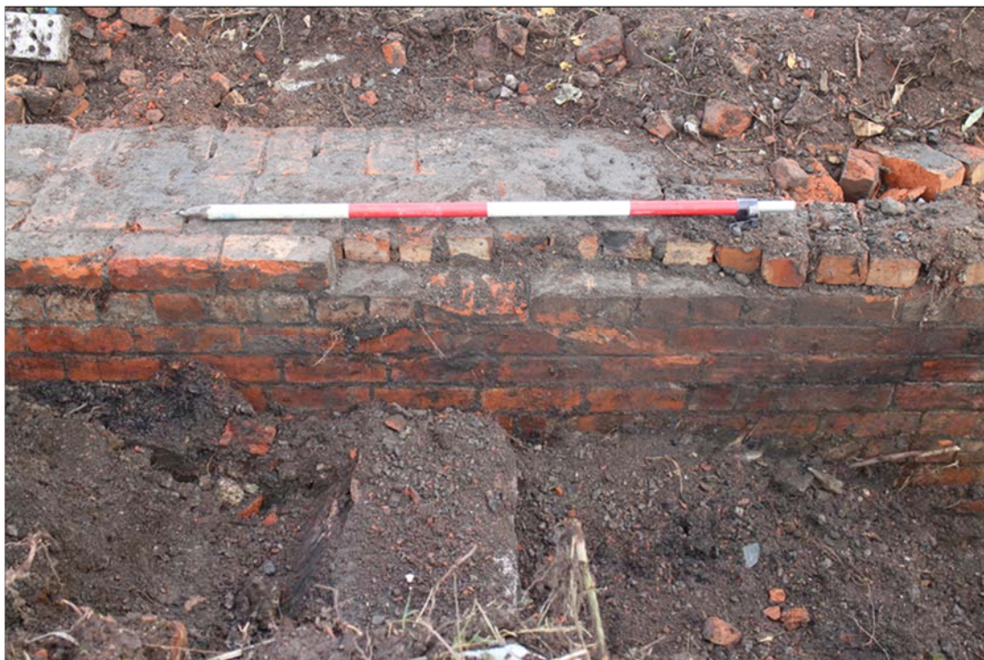
Plate 6: Wall 304 looking north-east, scale 2m
