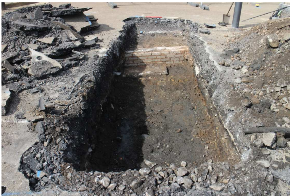
Plate 8: Trench 3 looking west, scale 1 x 1m
