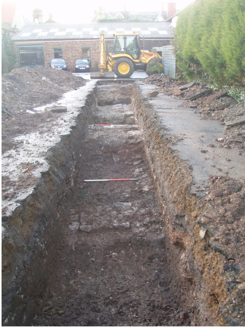
Plate 10: Trench 3; eastern end showing wall 325 in foreground and wall 320 along right side
