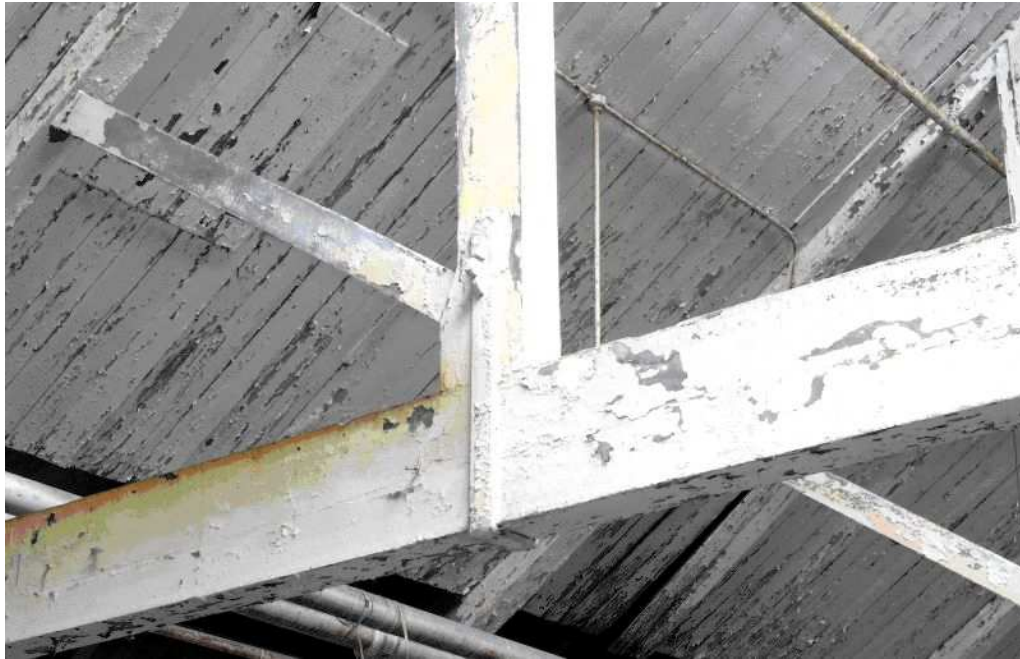
Plate 15: Detail of the bolted straps on the tie-beams
