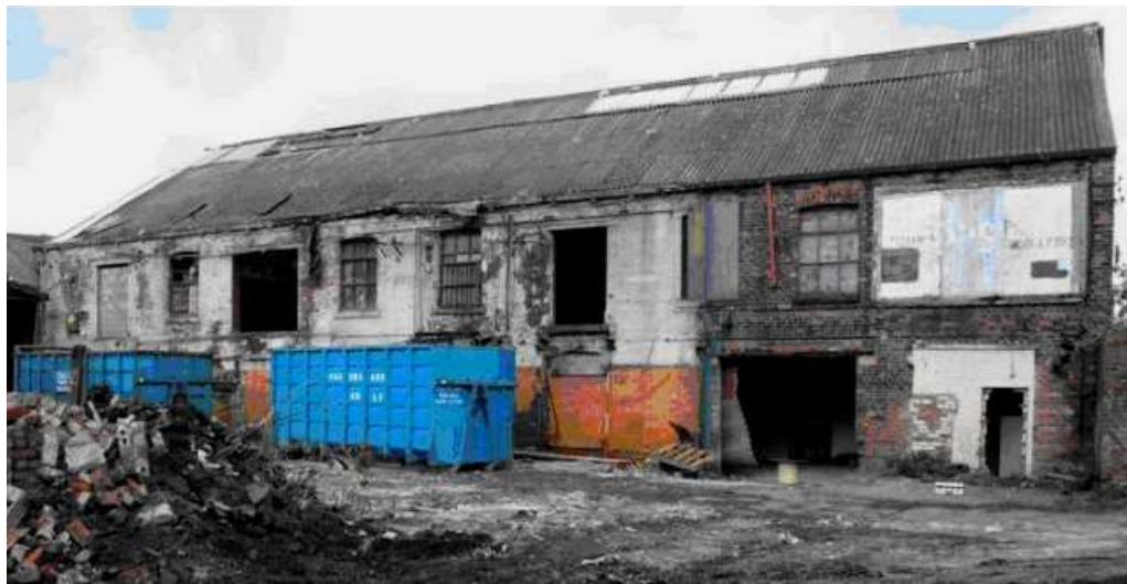
Plate 6: South-facing elevation of the building
