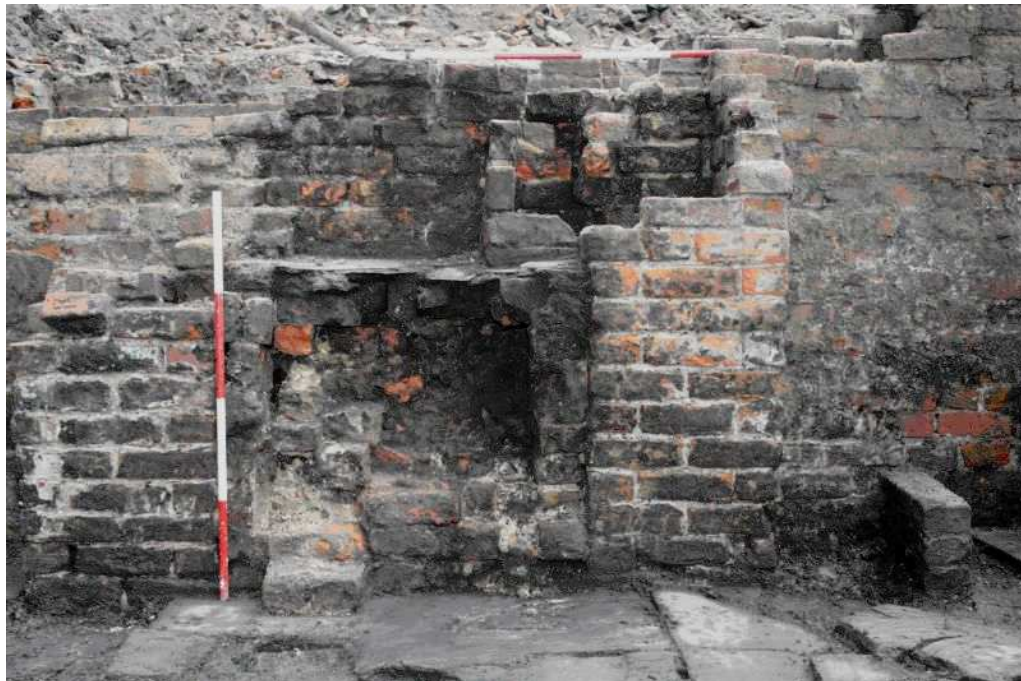
Plate 52: Fireplace within Room 7
