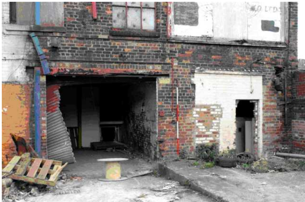
Plate 7: Entrance arrangement at the eastern end of the ground floor
