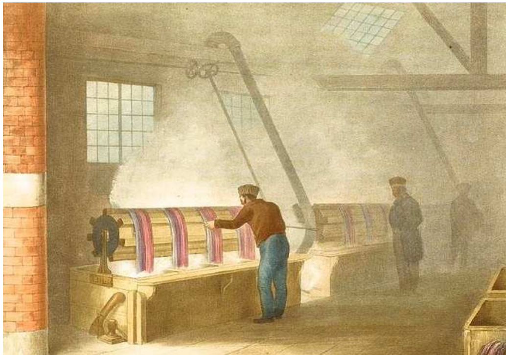
Plate 58: Steam-assisted dyeing technique in the 1840s (reproduced from Barfoot 1840)
