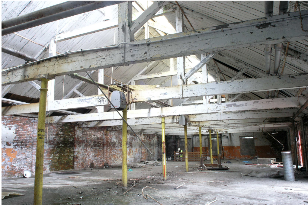
Plate 14: General view looking east across the first floor
