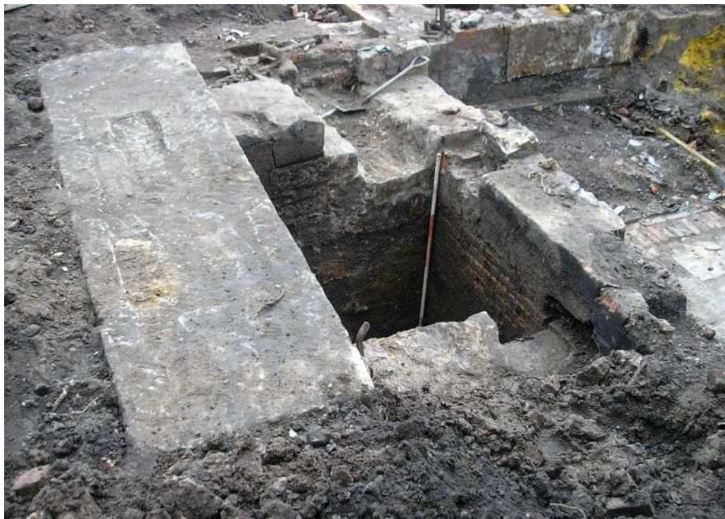
Plate 23: The foundations for a steam engine adjacent to the wash room, looking south-east
