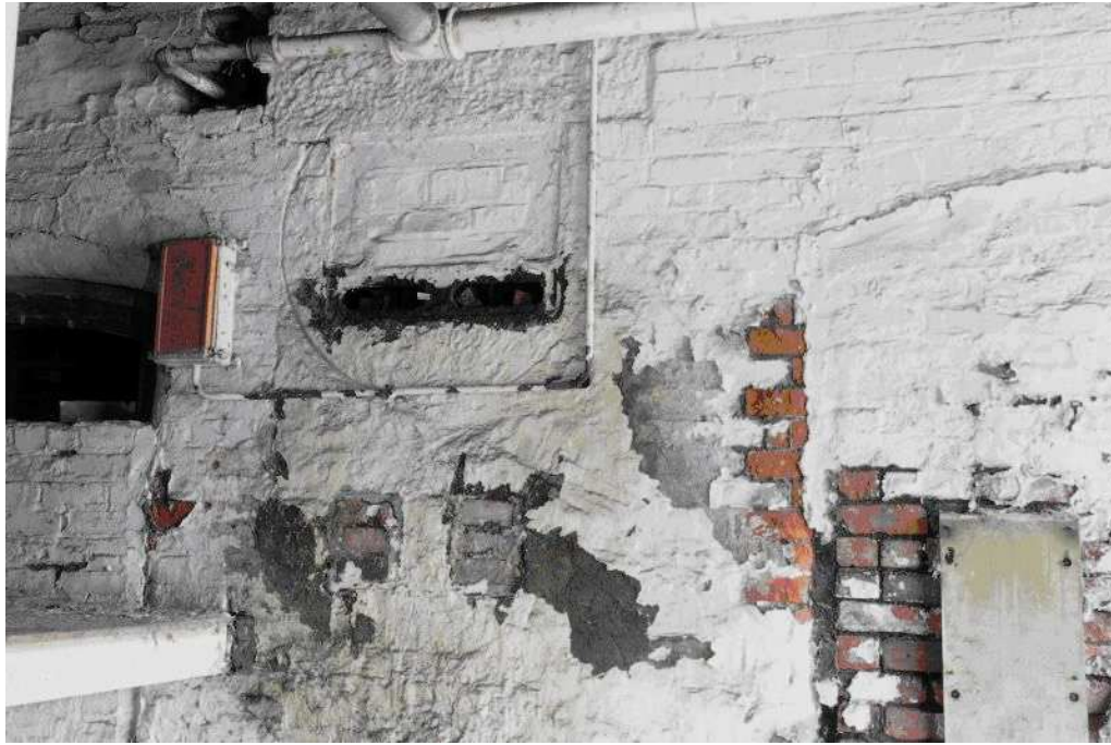
Plate 12: Detail of the in-filled central bearing-box, showing friction groove
