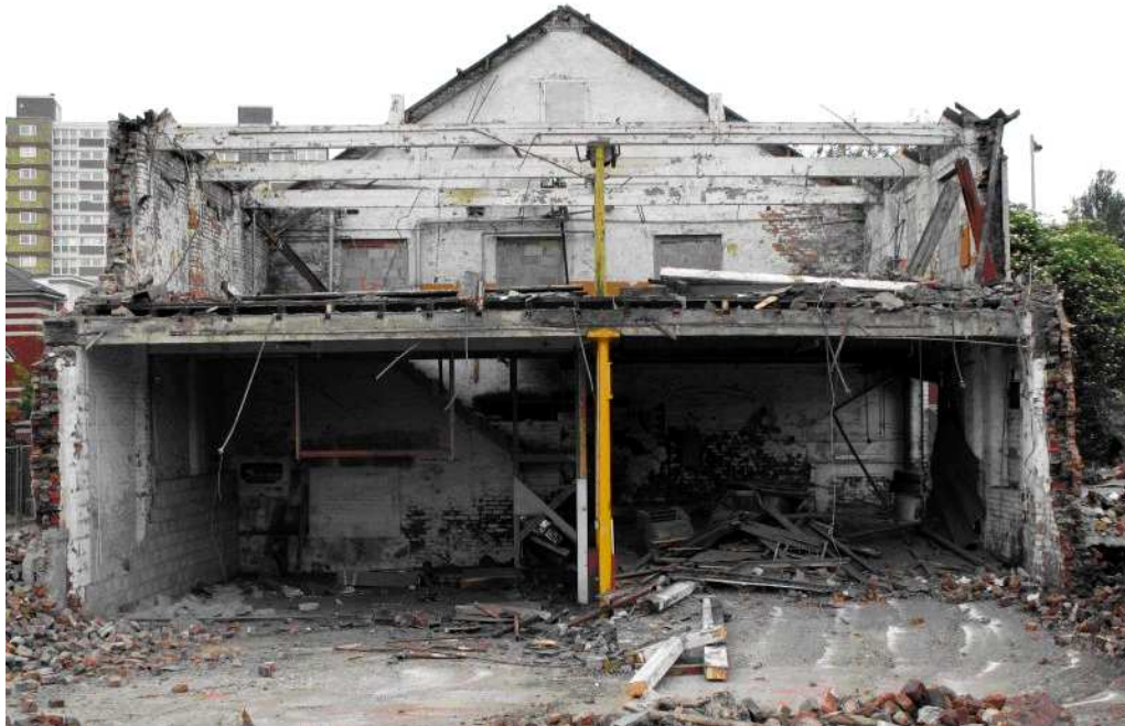
Plate 19: Cross-section of the building during demolition, looking east
