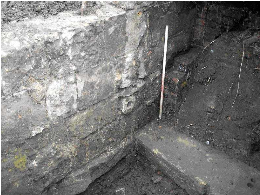
Plate 24: West wall of engine room 136 , showing the northern brick wall and sandstone block
