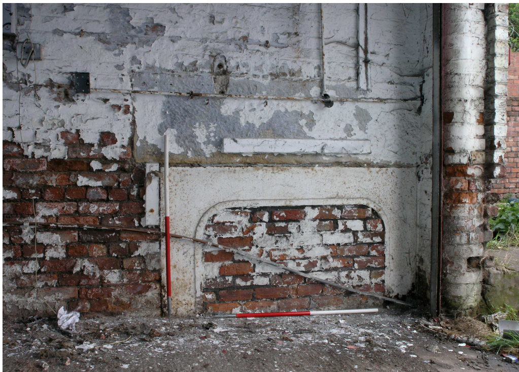
Plate 11: Detail of a primary transmission bearing box, in-filled with brick
