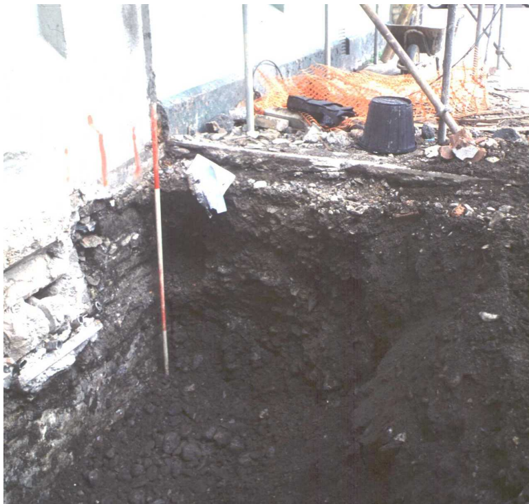
Plate 2: Post Office wall showing blocked chute, and west-facing section
