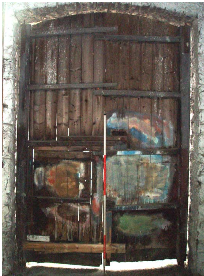
Plate 12: Detail of the internal face of the wagon door
