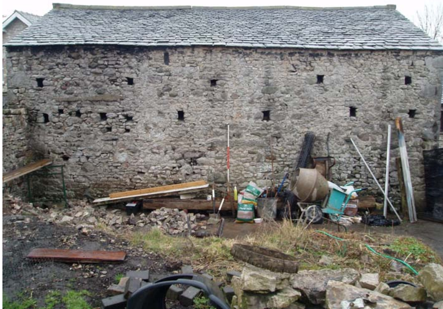
Plate 9: The south-east elevation, including evidence of an outshut at the north-west end
