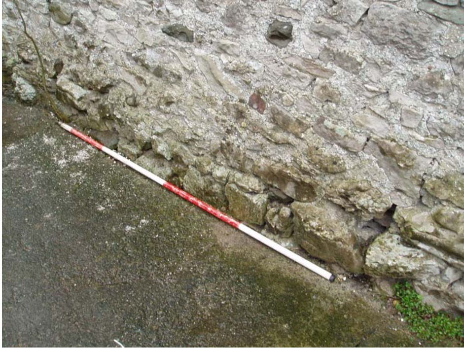
Plate 5: Detail of the foundation course on the south-west elevation
