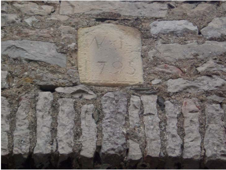
Plate 3: Detail of the re-used foundation stone above the wagon door
