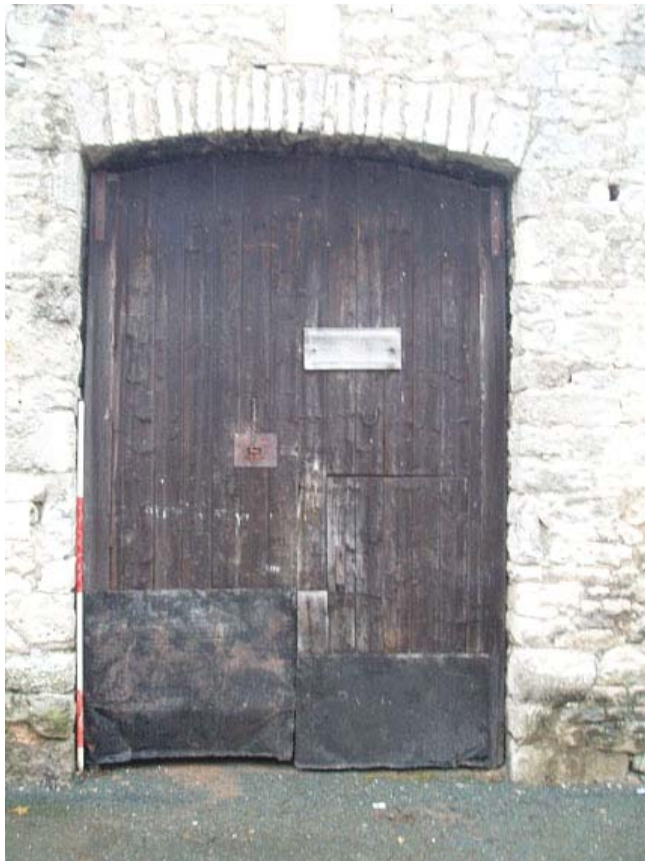
Plate 2: Detail of the wagon door on the south-east elevation
