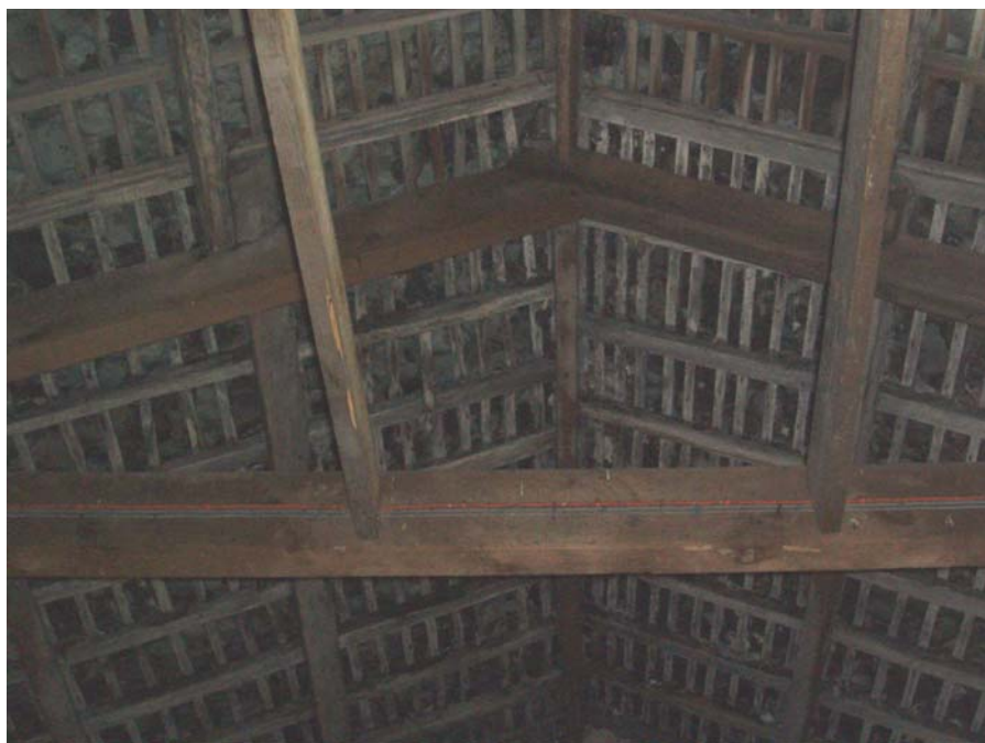
Plate 10: Detail of the north-east principal rafter truss
