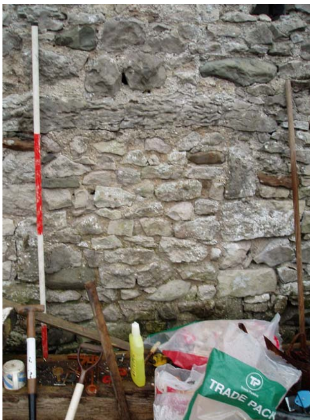
Plate 8: Detail of the blocked door on the north-west elevation
