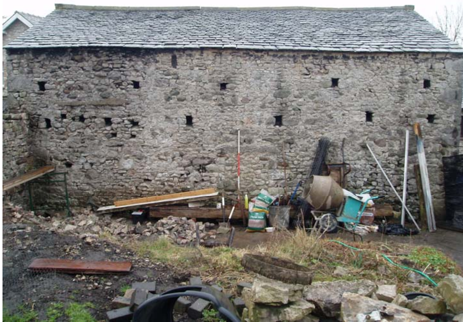
Plate 7: North-west facing elevation
