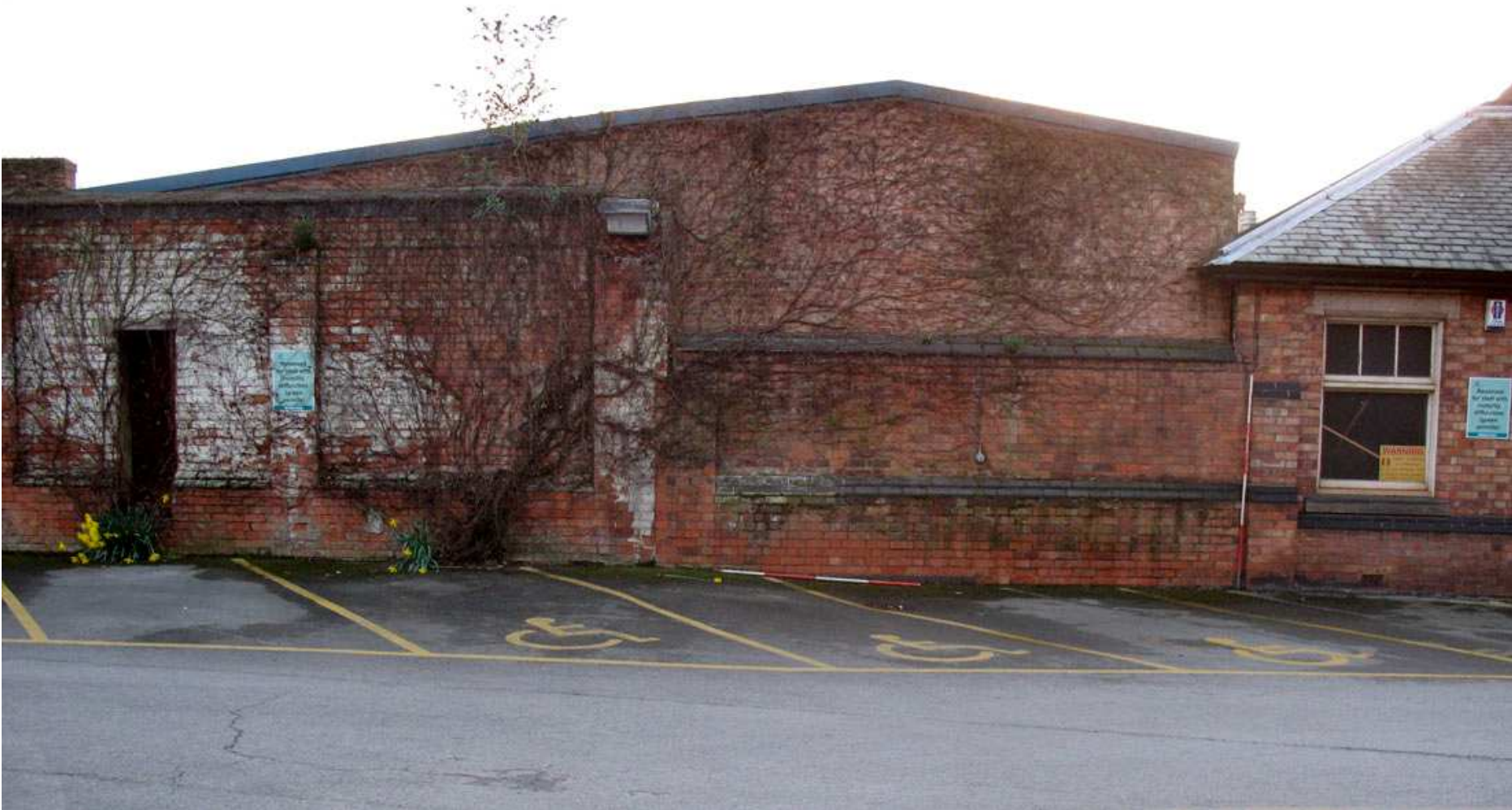
Plate 6: Photograph 4, north-western central section of the boundary wall
