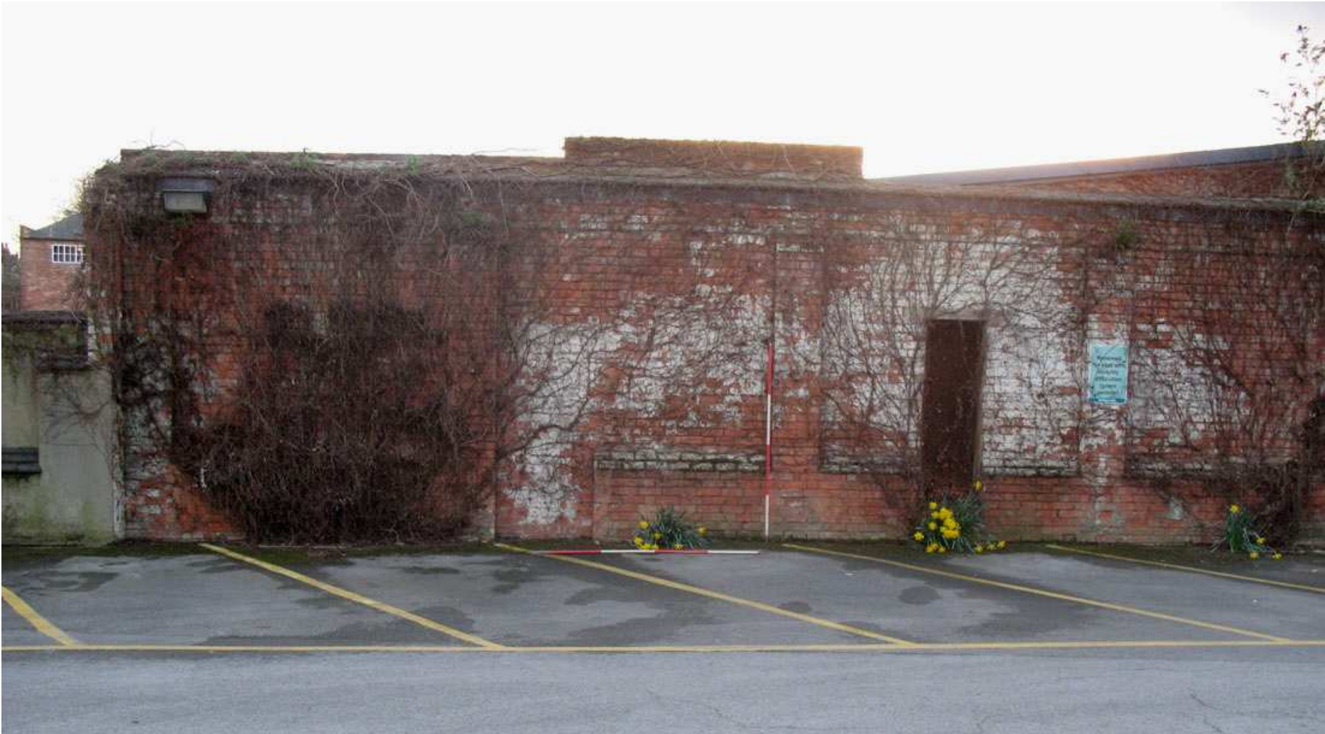
Plate 5: Photograph 3, central section of the boundary wall
