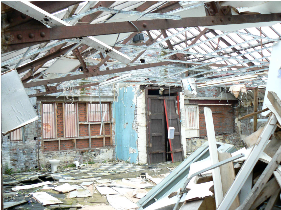
Plate 9: The hoist and taking-in doors against the rear internal elevation of 14 Great Moor Street
