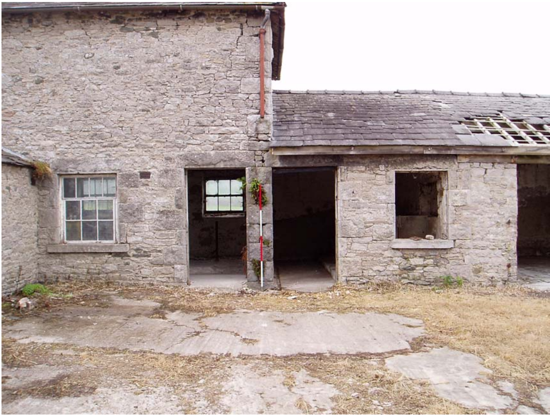
Plate 8: The west elevation (courtyard) of the east range, to the north
