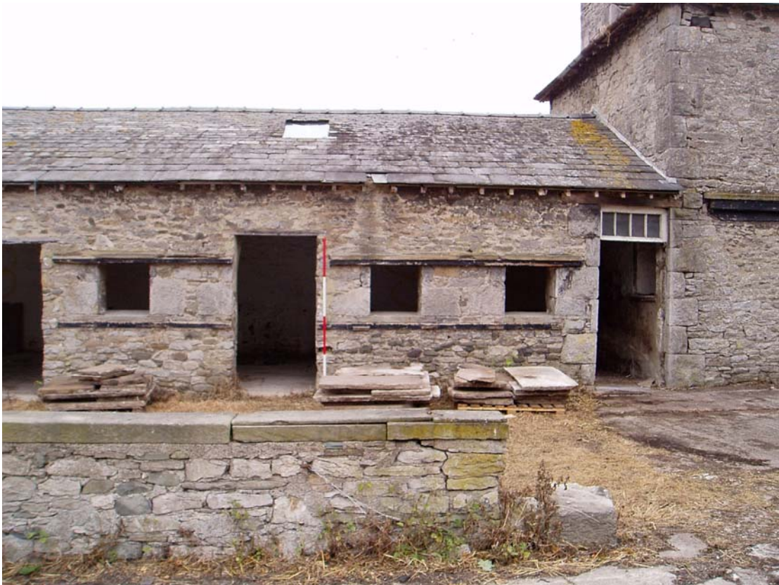
Plate 9: The east elevation (courtyard) of the west range, to the north
