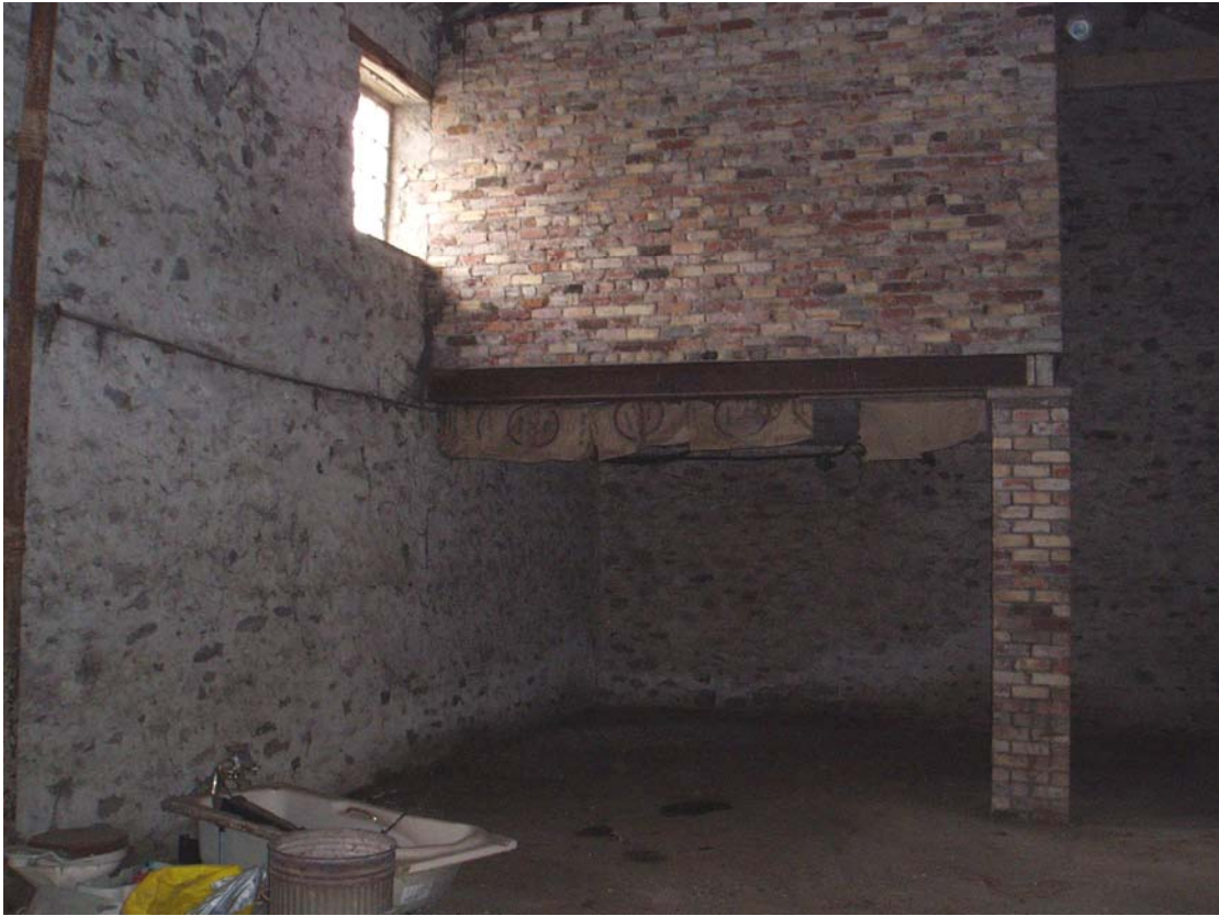
Plate 16: The brick extension of the cottage within the barn
