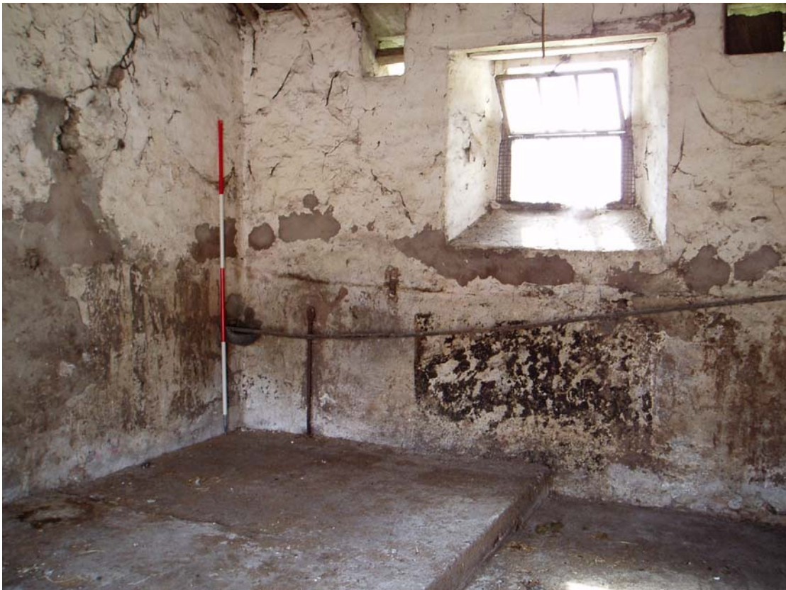
Plate 19: General view of room 13
