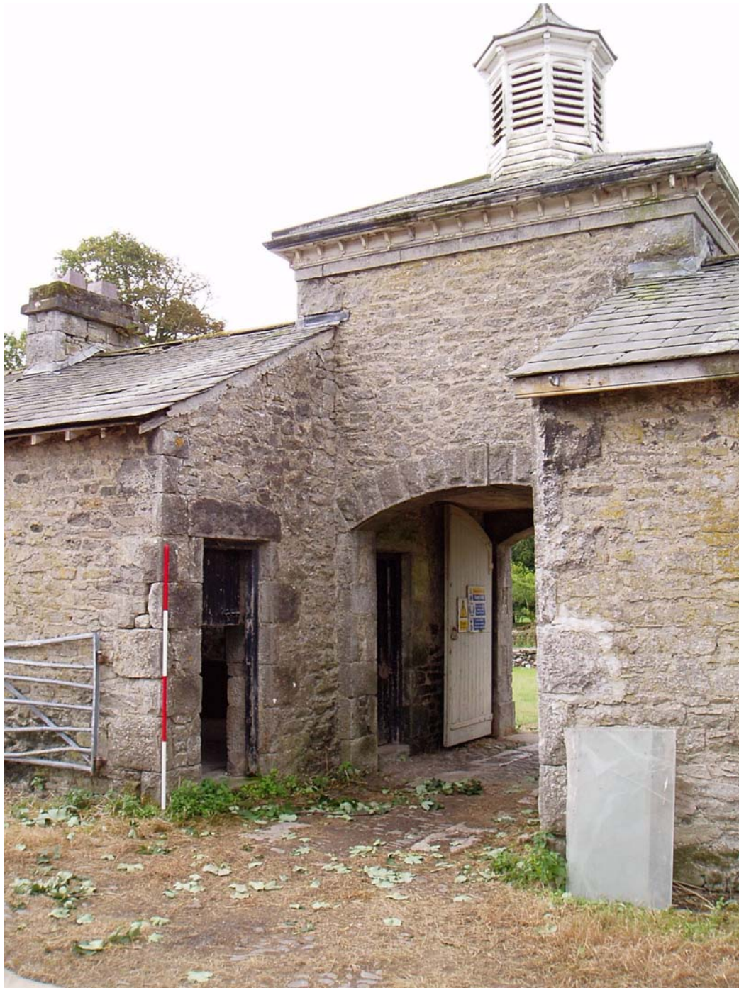
Plate 10: The rear of the clock tower (courtyard) and the south range
