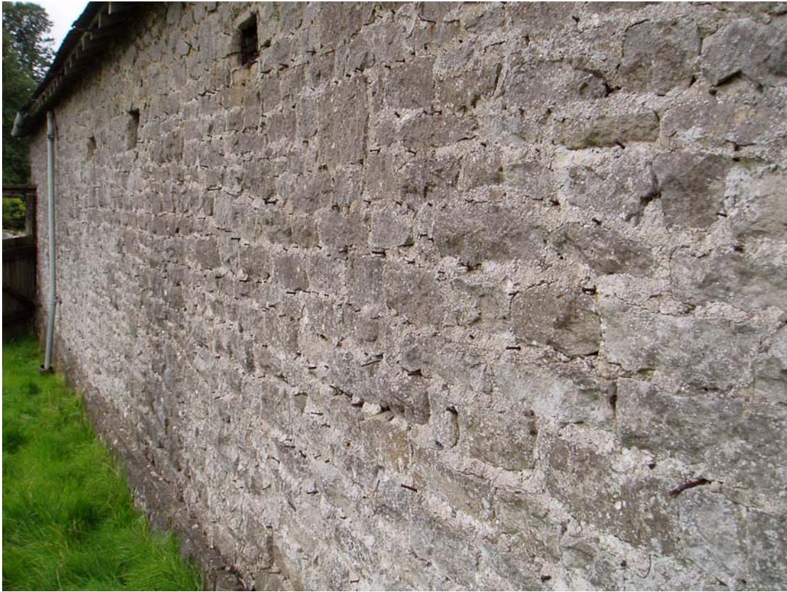
Plate 11: Detail of the iron nails on the east wall of the east range
