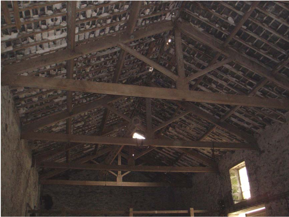
Plate 13: The king post trusses in the barn
