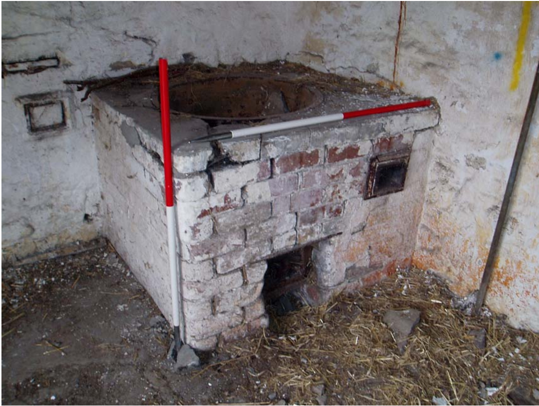
Plate 22: The washpot in room 4, with the blocked flue to the left
