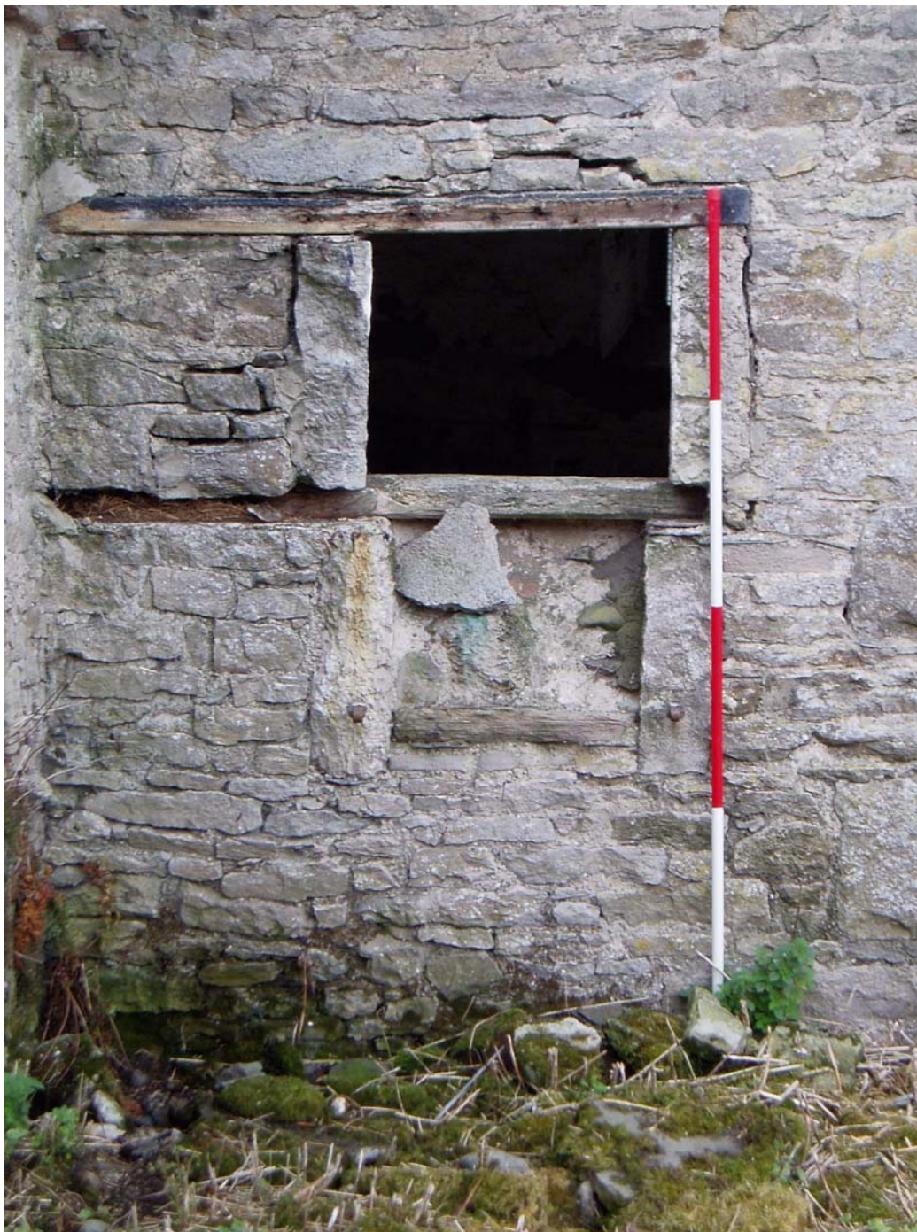
Plate 15: Detail of the partially blocked window on the east extent of the south range (courtyard)
