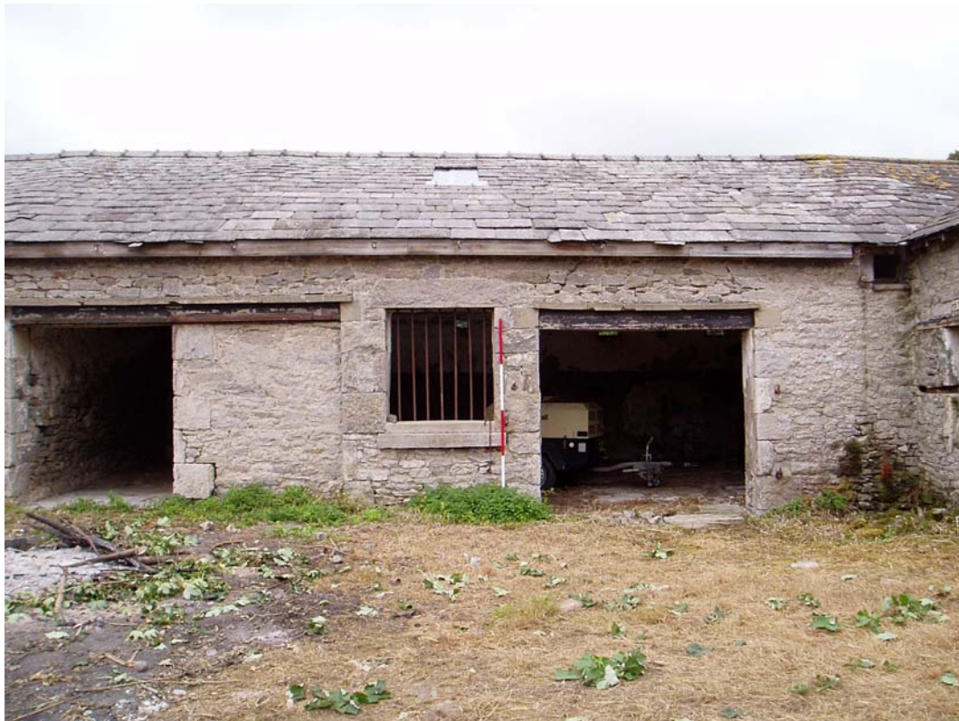
Plate 7: The west elevation (courtyard) of the east range, to the south
