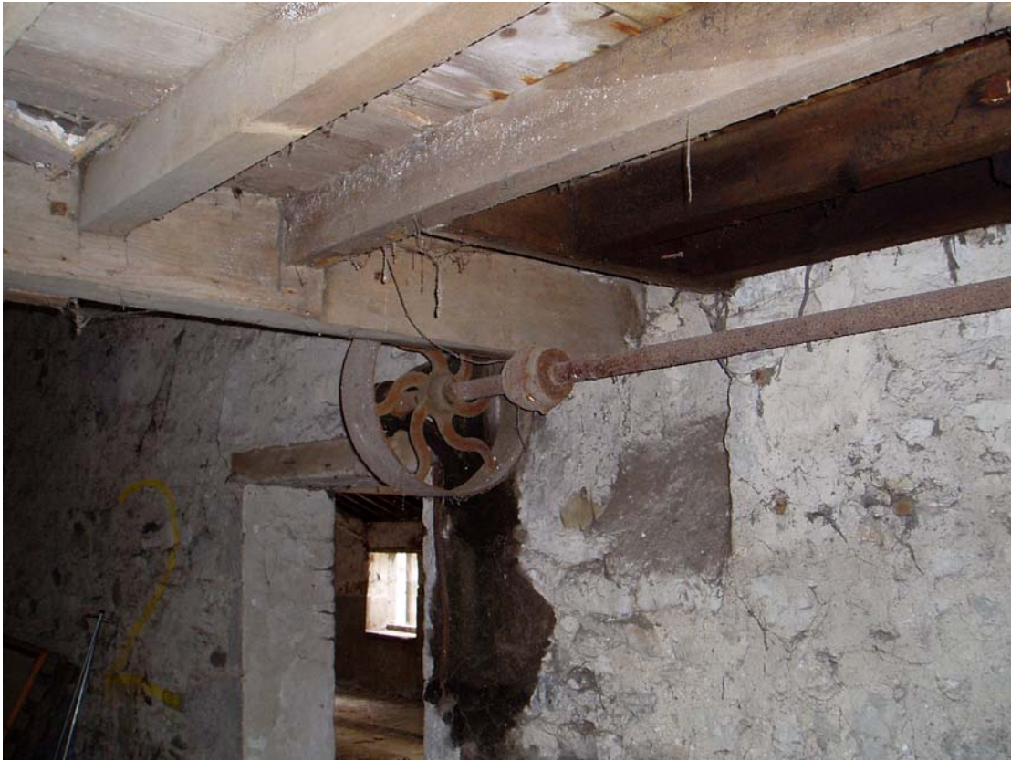
Plate 18: South-east-facing view of the lineshaft and spoked flywheel
