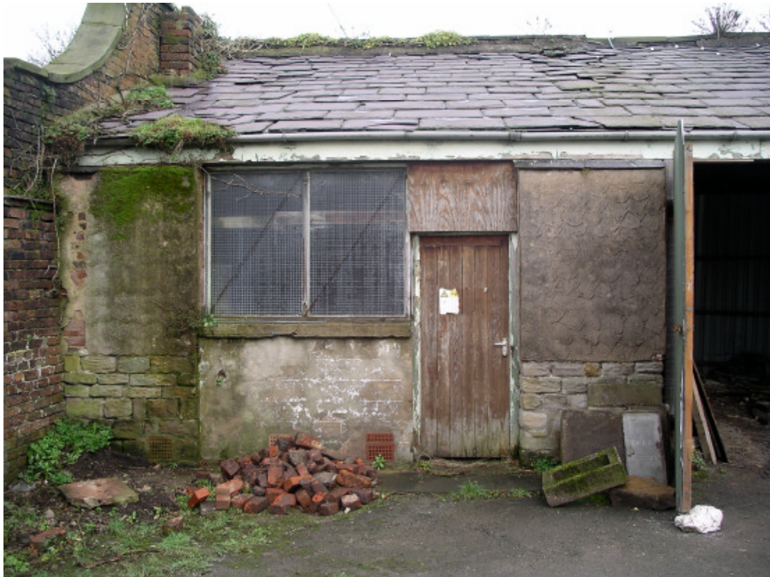
Plate 4: The outbuilding abutting the orchard garden wall (Site 33), looking north
