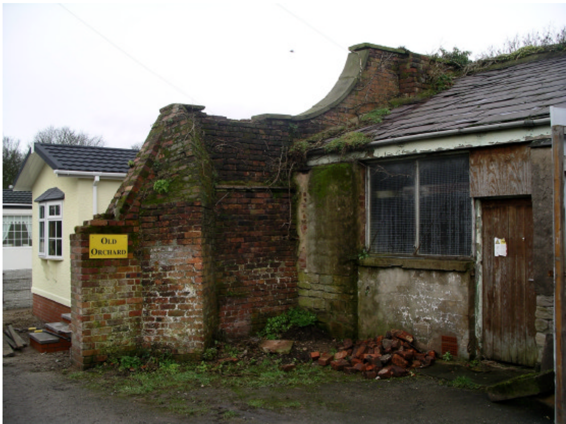
Plate 2: The north side of the entrance to the orchard garden (Site 33), looking north-west
