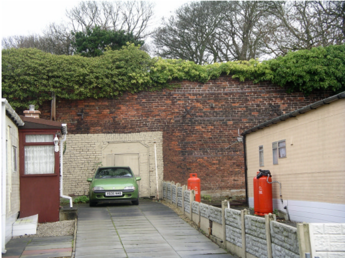
Plate 1: The orchard garden wall (Site 33), looking north
