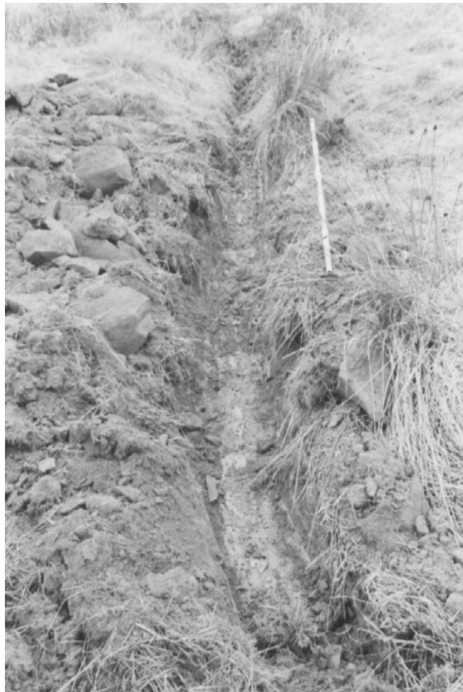
Plate 4: Excavation for insertion of pipe into drainage ditch, looking south
