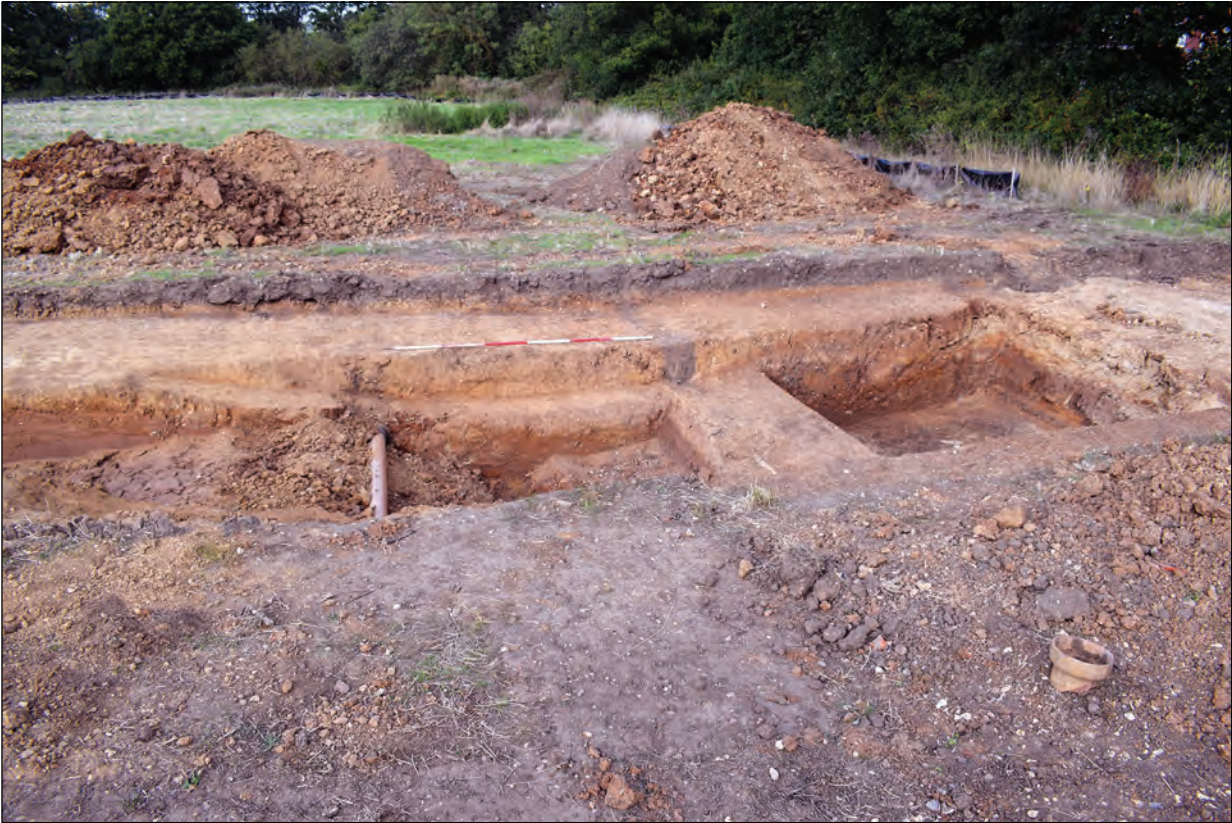
Plate 5: Area 2, excavation trench from the south (after further machine excavation)
