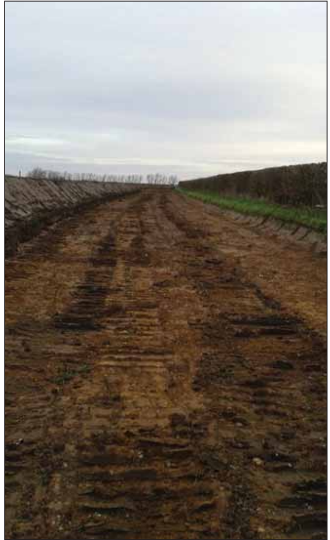
Plate 2: Site 6 topsoil strip, looking north north-east
