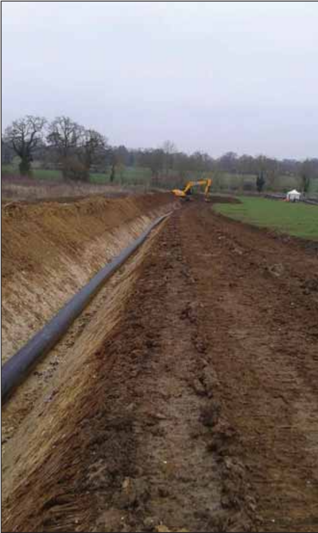
Plate 1: Site 3 topsoil strip and pipe trench looking north-west
