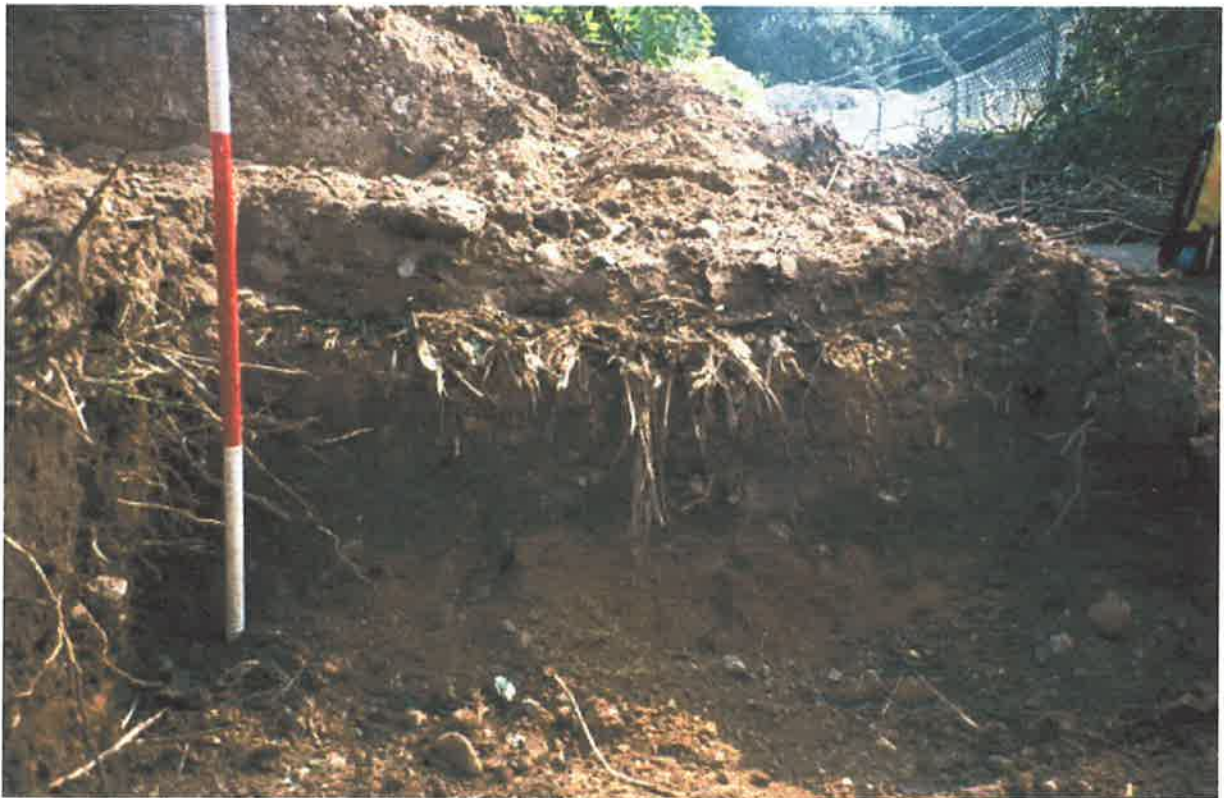
Plate 2: Manhole pit 1, west-facing section
