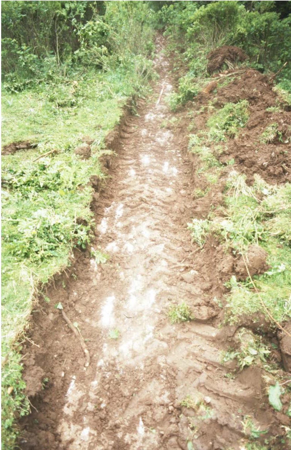
Plate 3: General view of evaluation trench looking north-east
