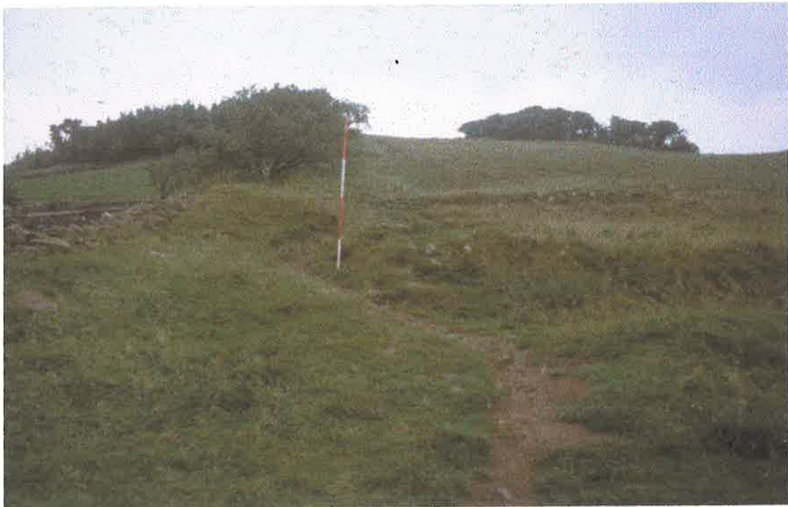
Plate 4: South-West Bank of the Milecastle Showing line of Erosion, Looking North-East
