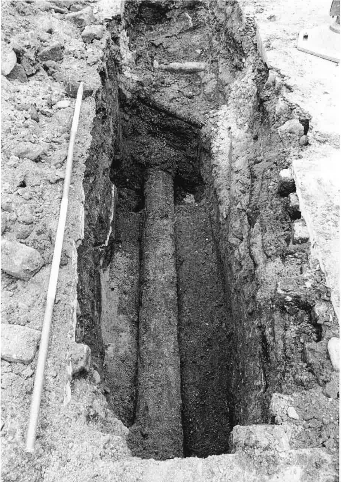
Plate 1: View of a typical trench showing original water pipe at base
