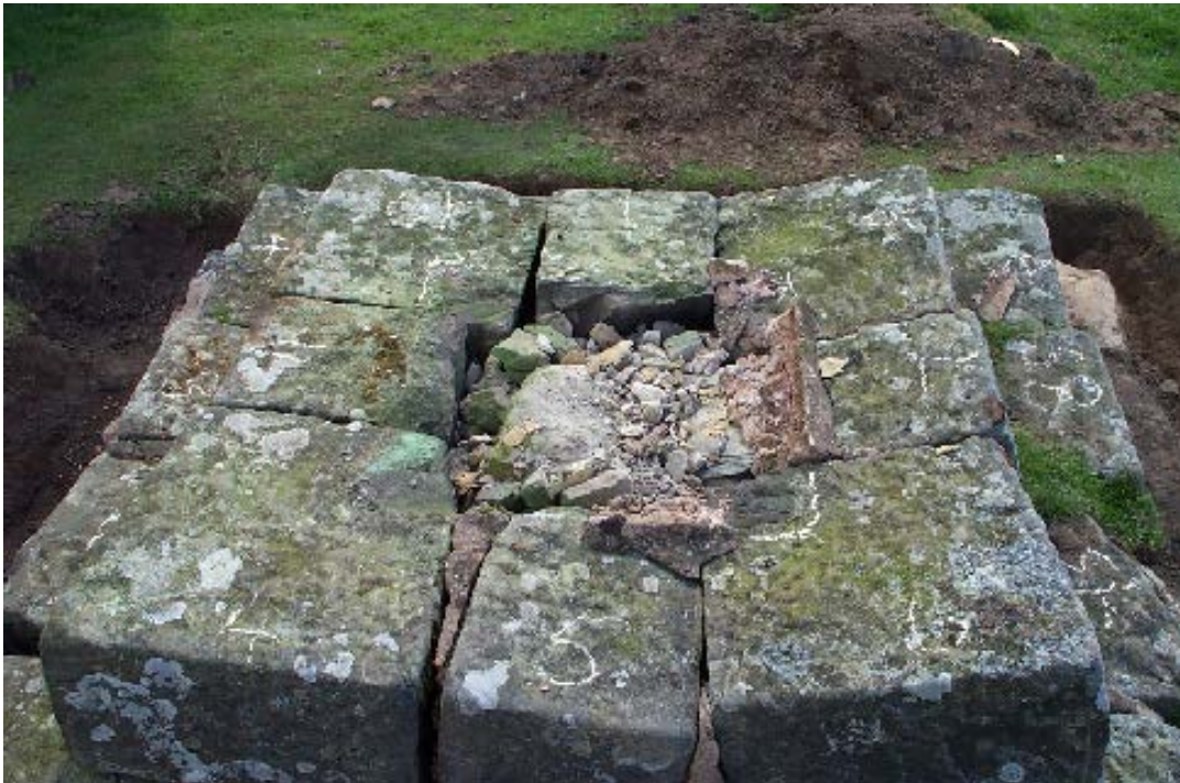
Plate 6: The rubble core exposed
