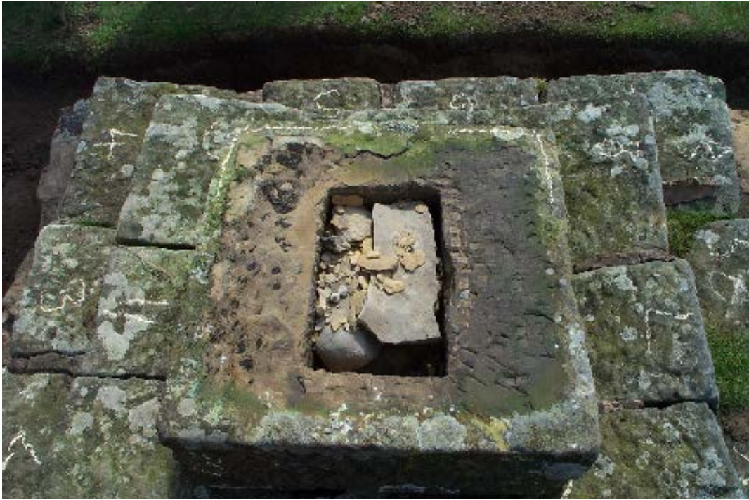
Plate 5: Rubble core through the hollow pillar base
