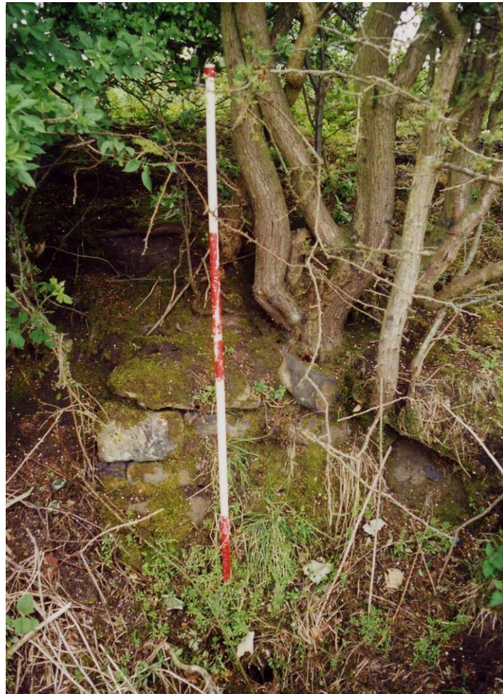
Plate 2: Site 08, Garswood-Pewfall Incline, sectional view, looking North
