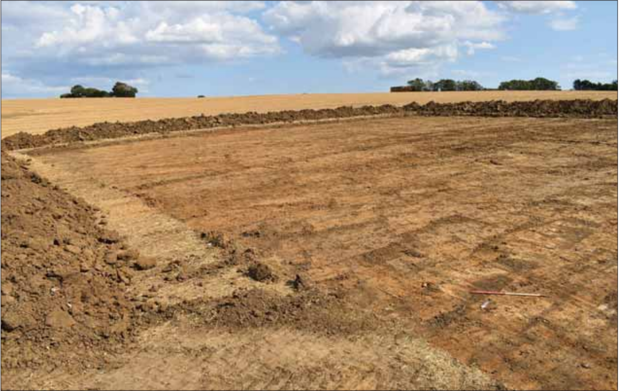
Plate 3: Compound area stripped, looking southeast.
