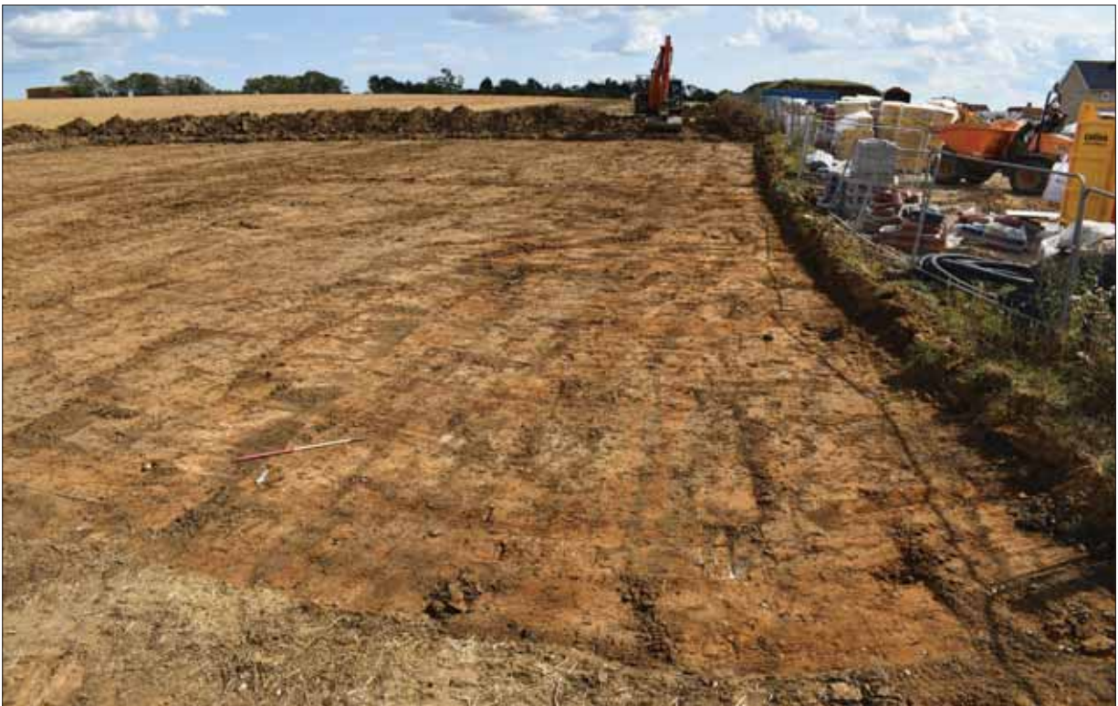
Plate 2: Compound area stripped, looking south.
