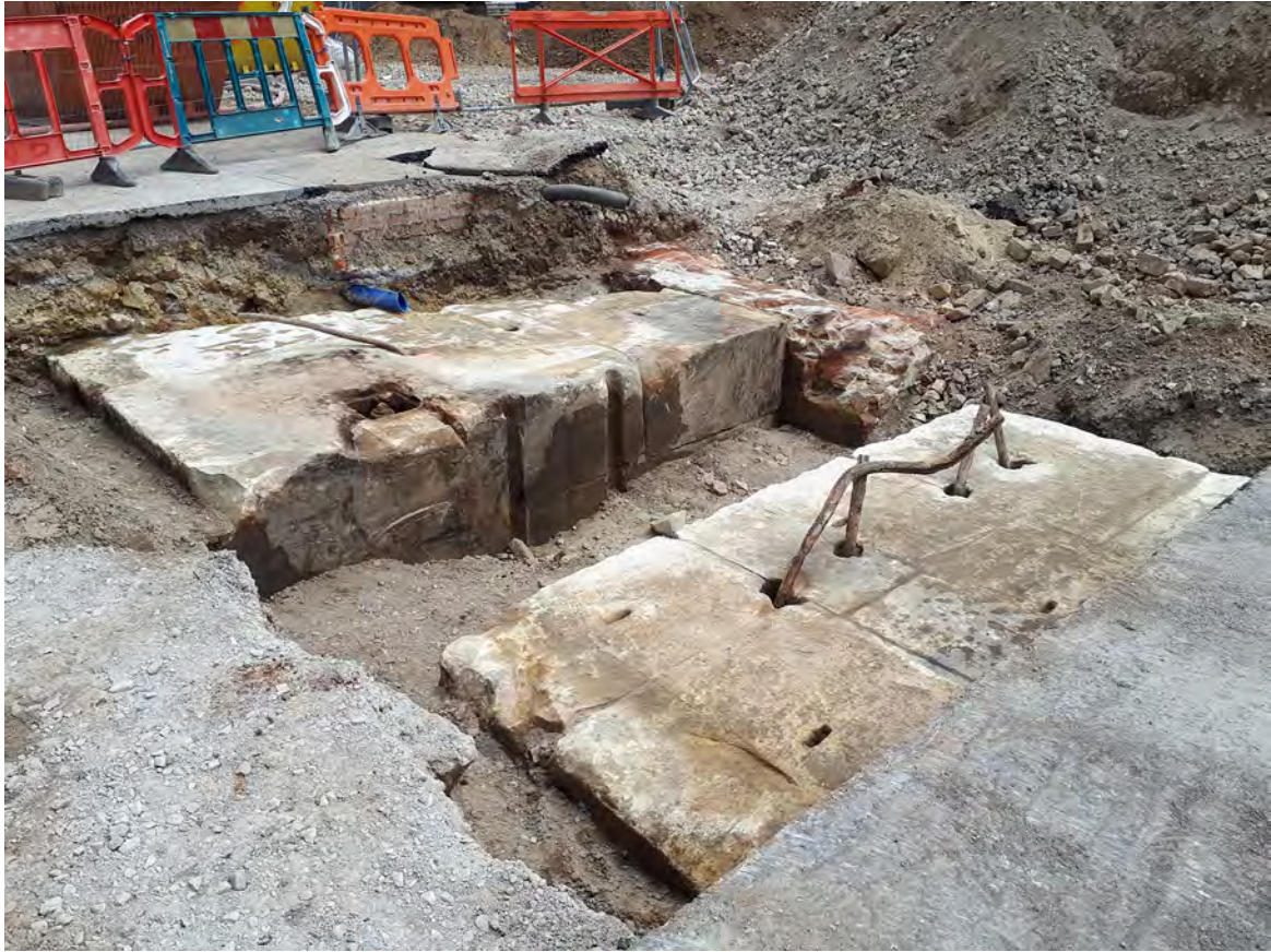
Plate 8: Stone structures 20187 and 20189, brick wall 20190, view to SW
