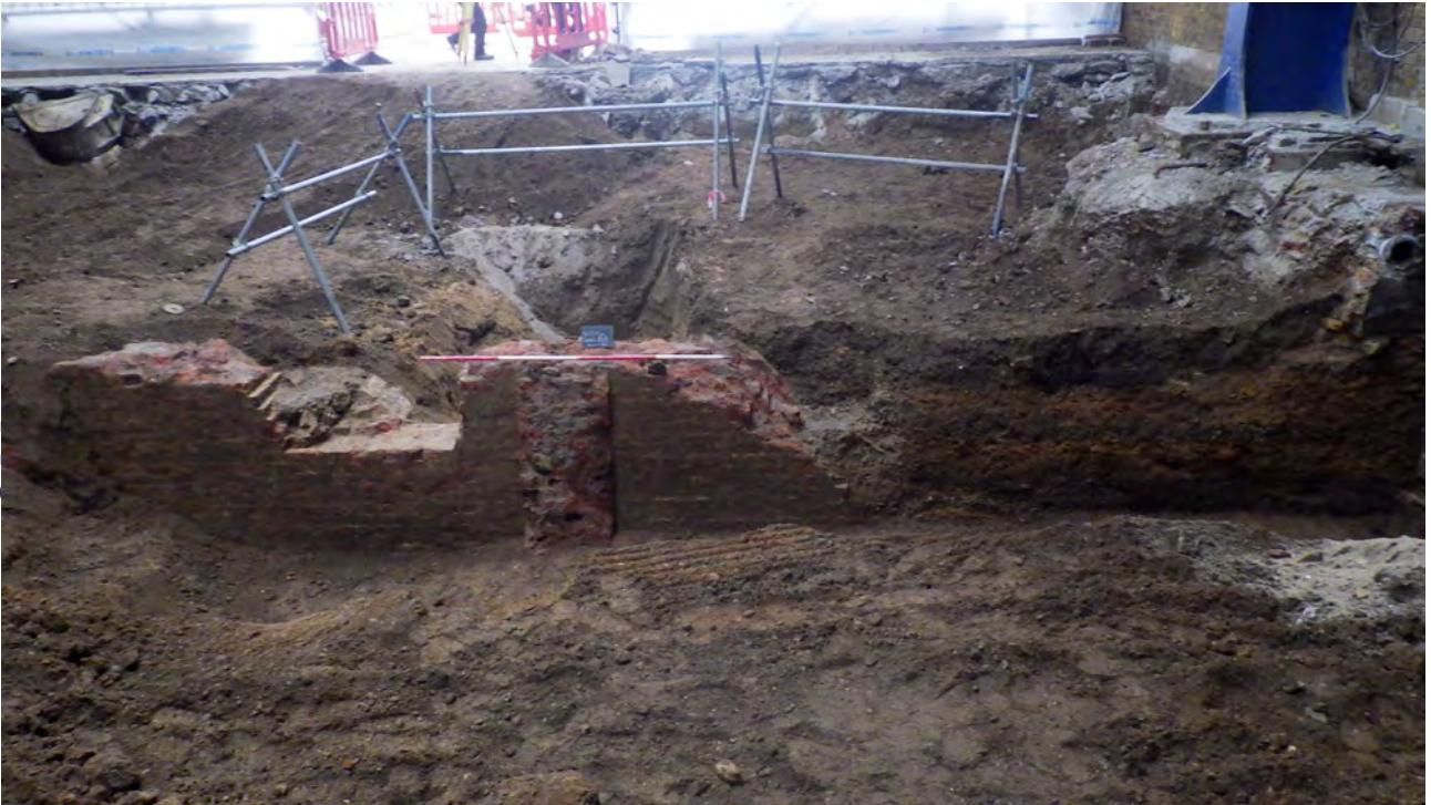
Plate 6: Wall 20150, view to E
