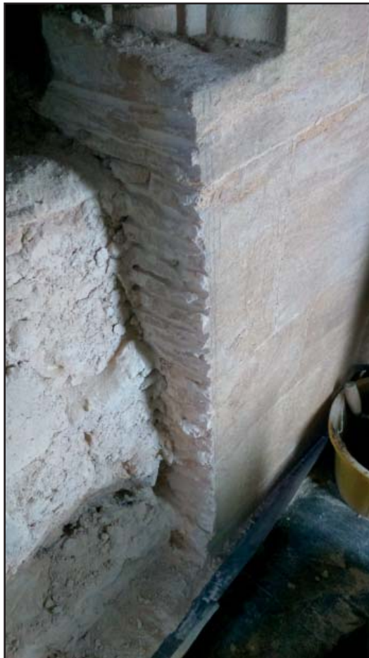
Plate 20: Detail of first floor window showing depth of worked stone and rubble core
