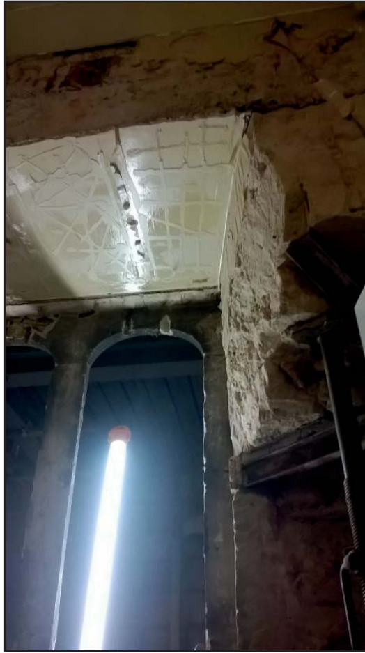
Plate 19 : First floor window following removal of modern material
