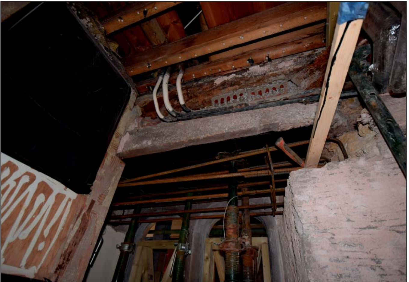
Plate 17: Second floor window following removal of modern material
