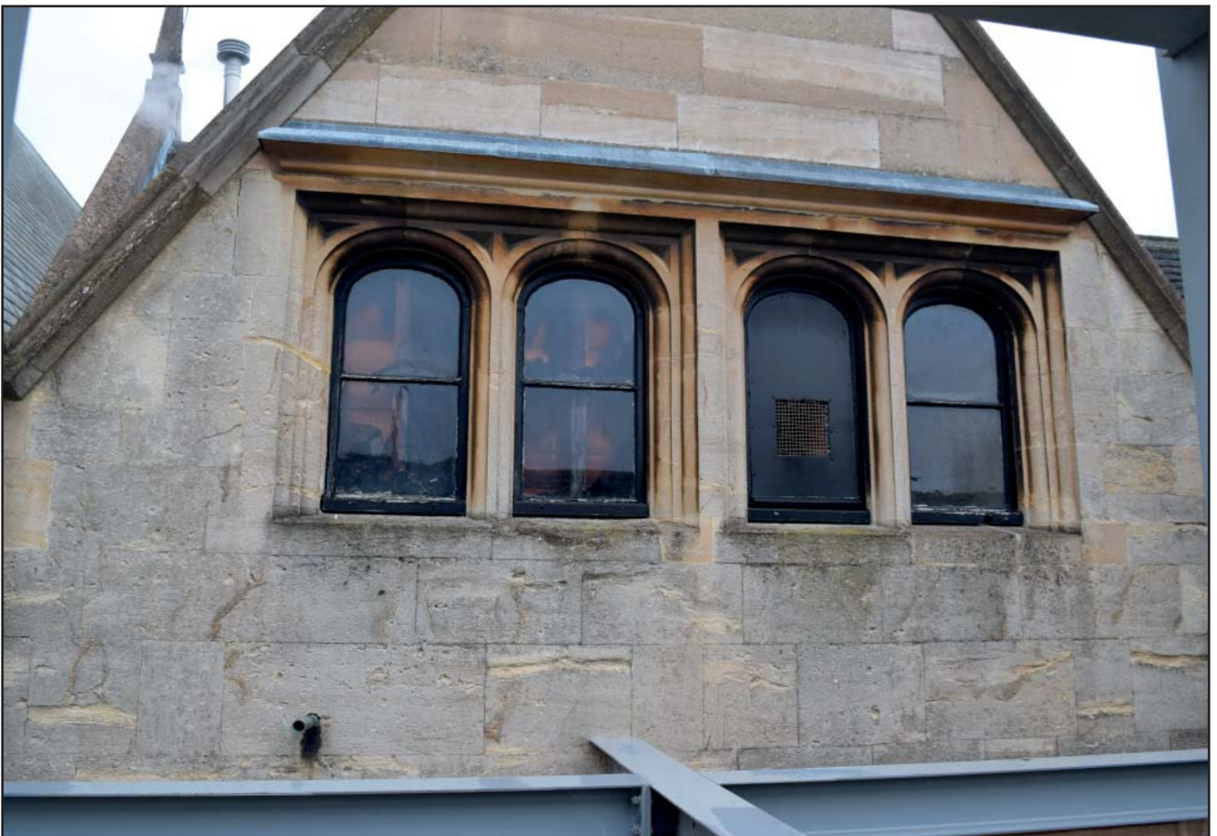
Plate 6: View of third floor windows
