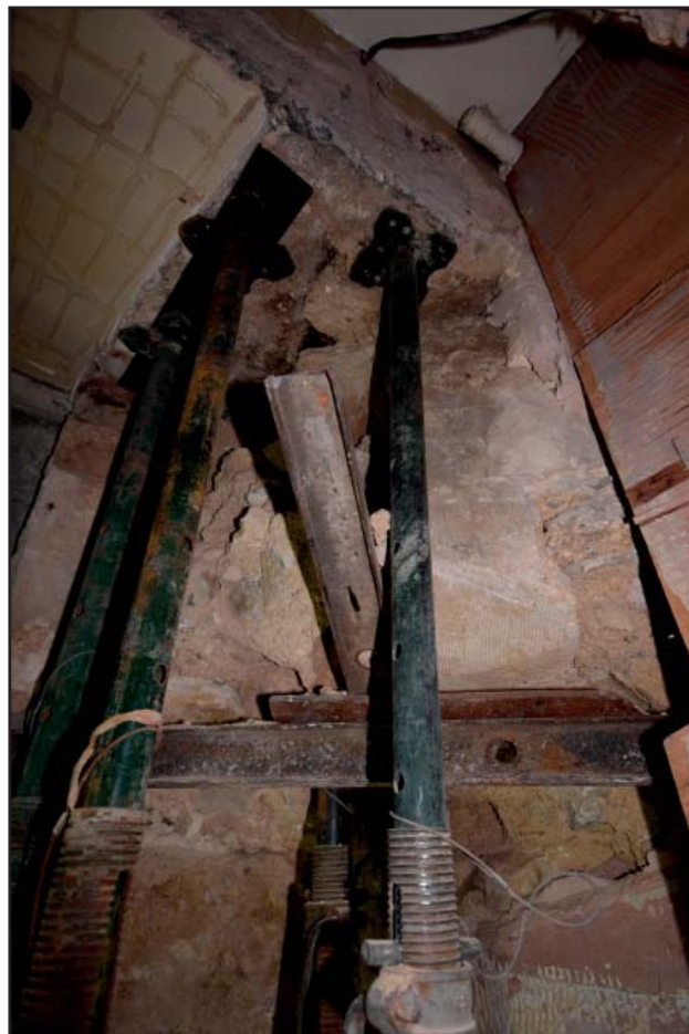
Plate 18: First floor window following removal of modern material
