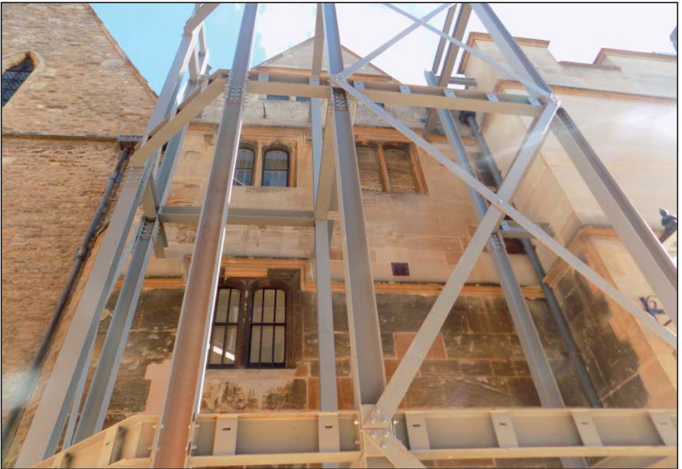
Plate 1: External view of first, second and third floor windows after extension frame constructions
