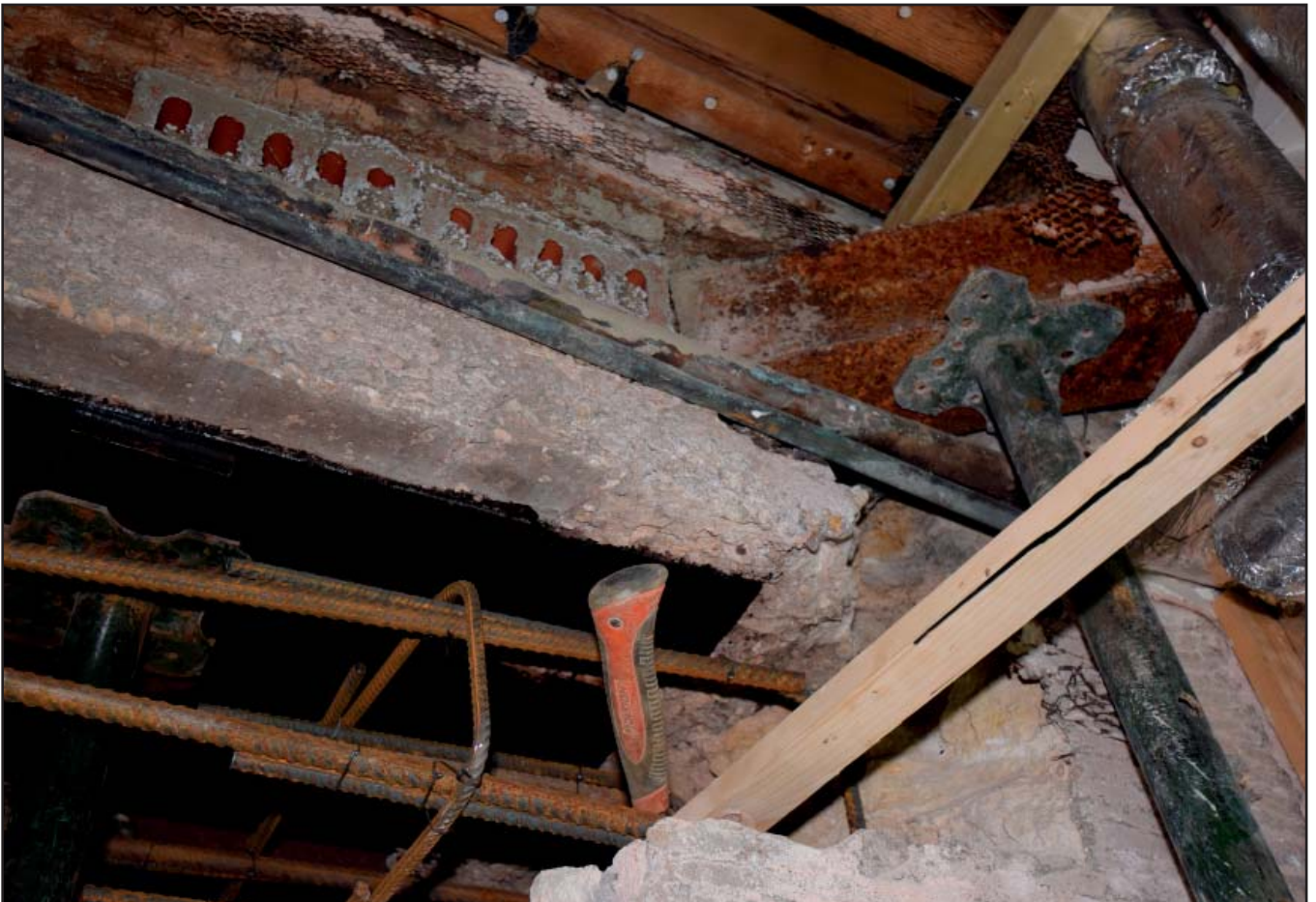
Plate 16: Second floor window following removal of modern material
