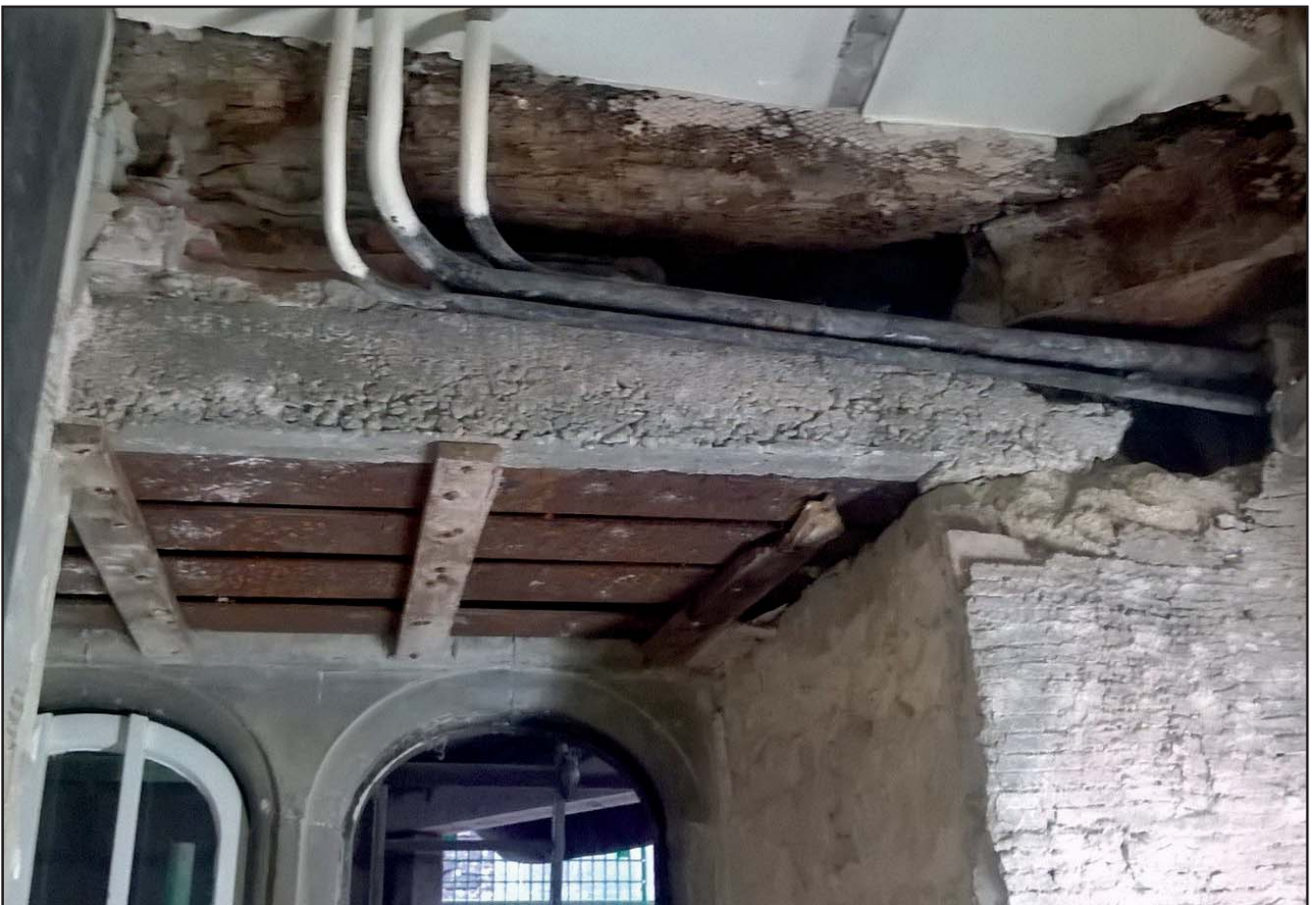
Plate 14: Second floor window following removal of modern material
