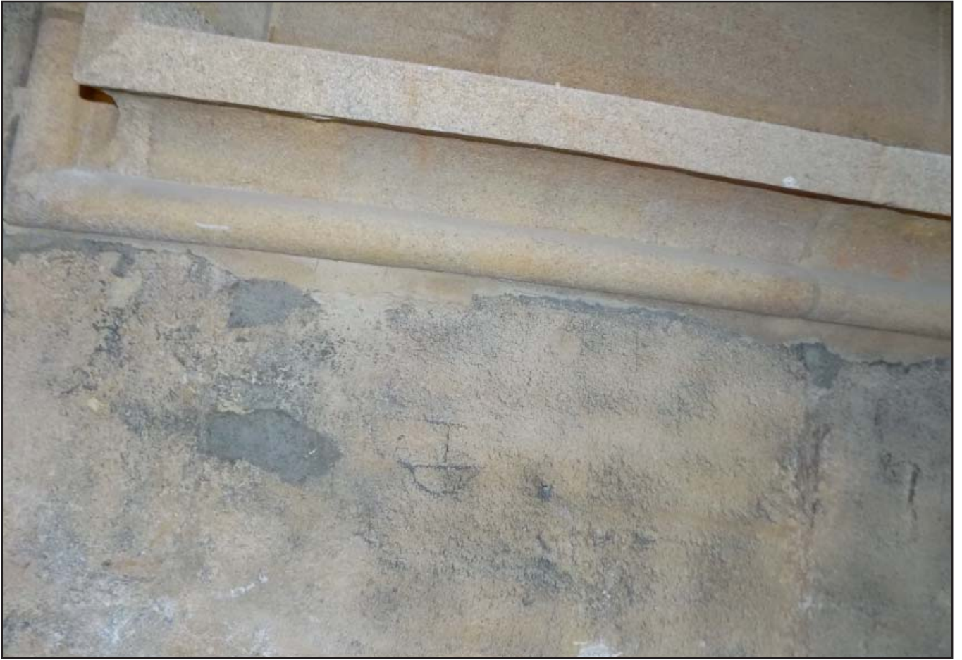
Plate 23: Detail of masons mark on 2nd floor of external elevation
