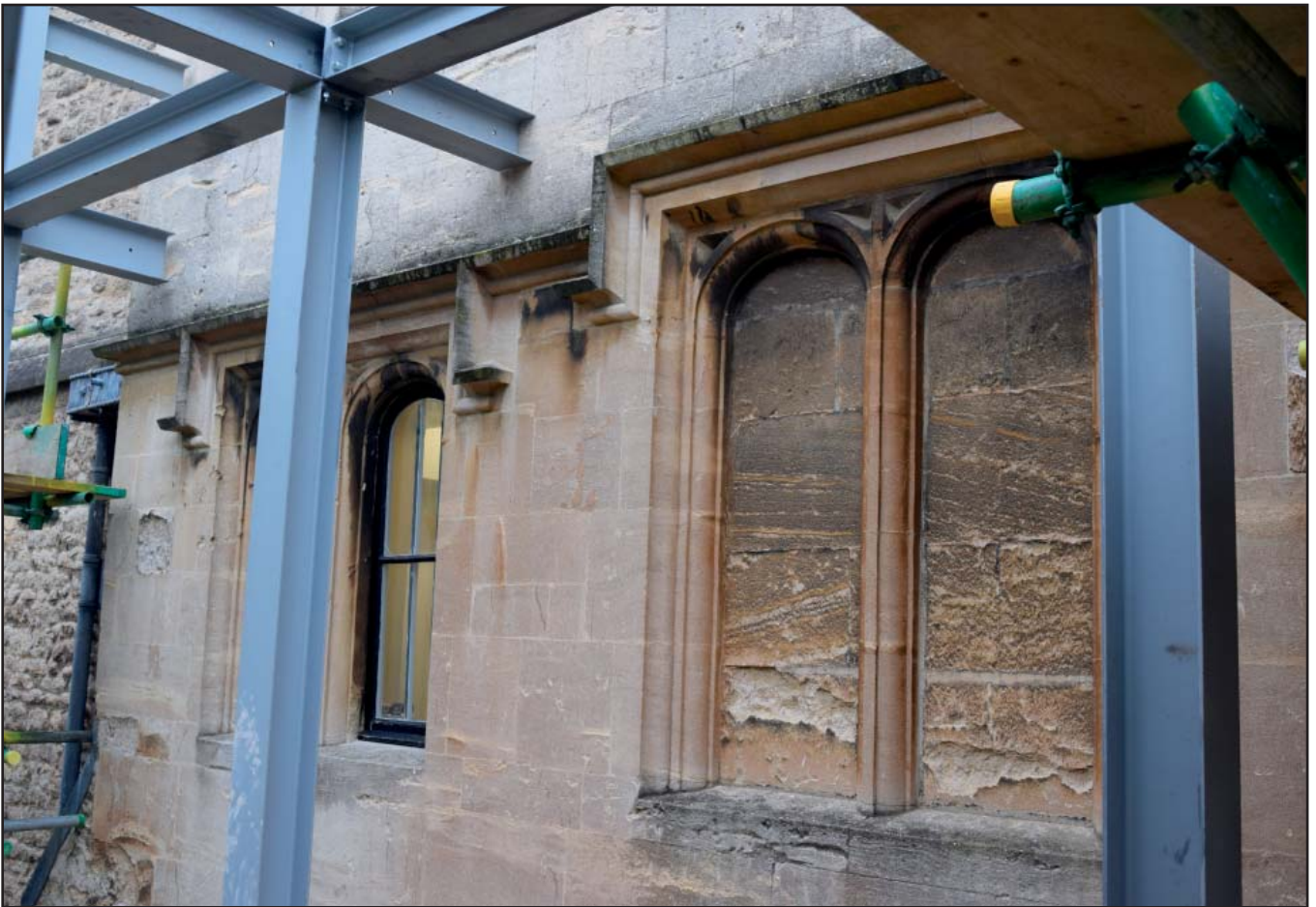
Plate 5: View of second floor windows
