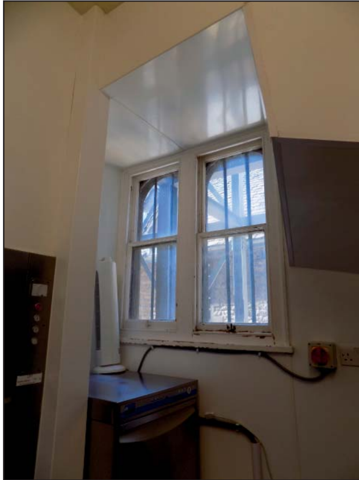
Plate 7: Internal view of first floor window
