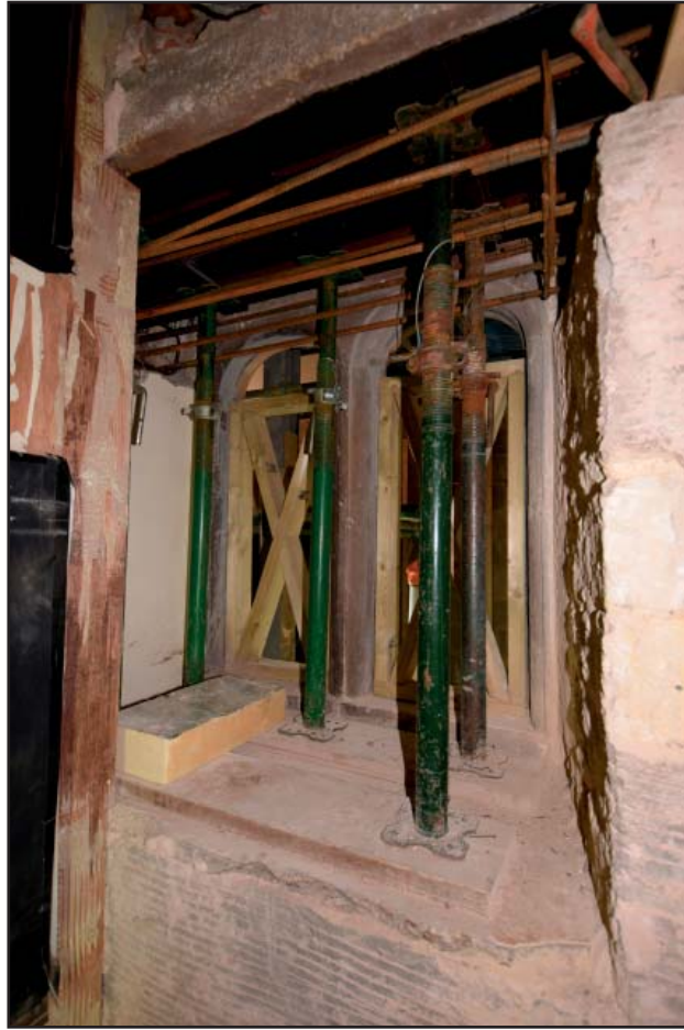
Plate 15: Second floor window following removal of modern material
