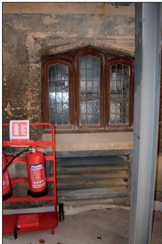
Plate 2: View of ground floor window inserted into former corridor opening to Mob Quad in 1960
