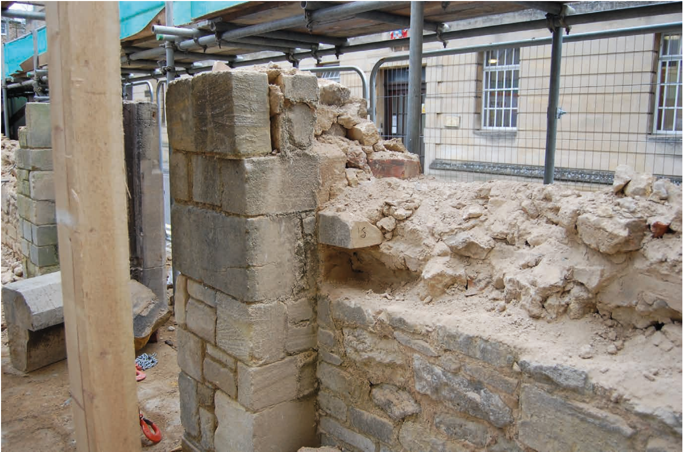
Plate 9: Inserted 19th century doorway in OA 103, looking north west
