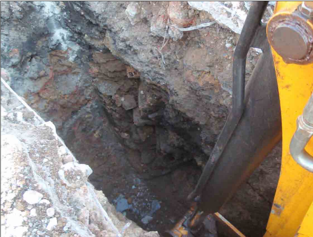
Plate 5: Wall in Test Pit 19
