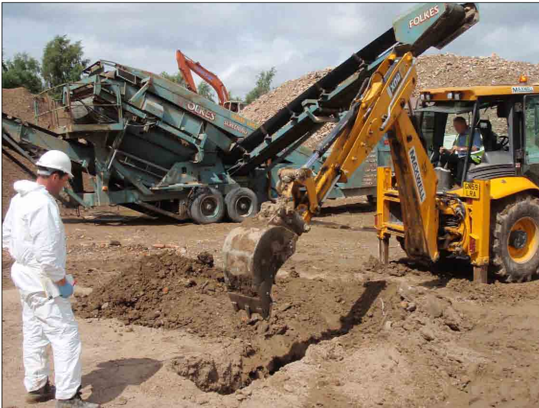
Plate 3: Machining of Test Pit 20
