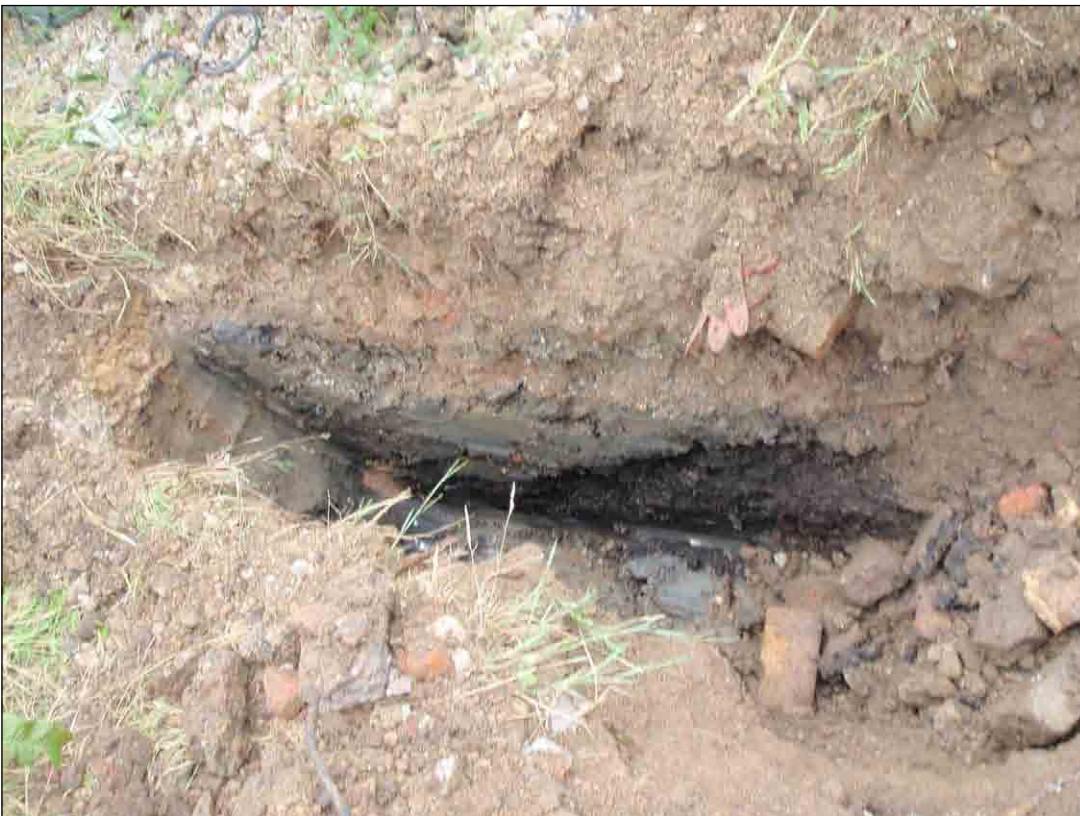
Plate 6: Pit in Test Pit 23
