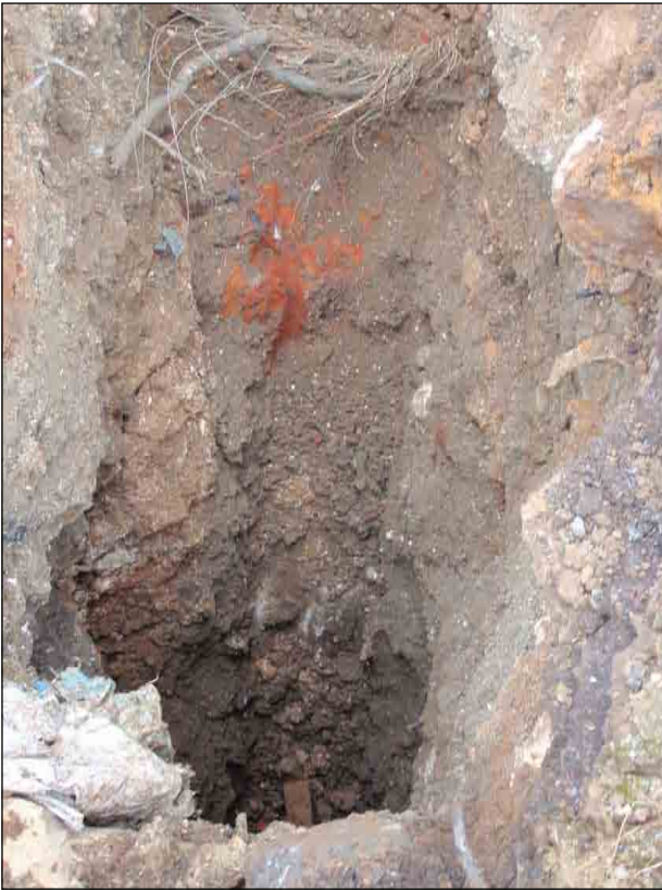
Plate 7: Wall in test Pit 24
