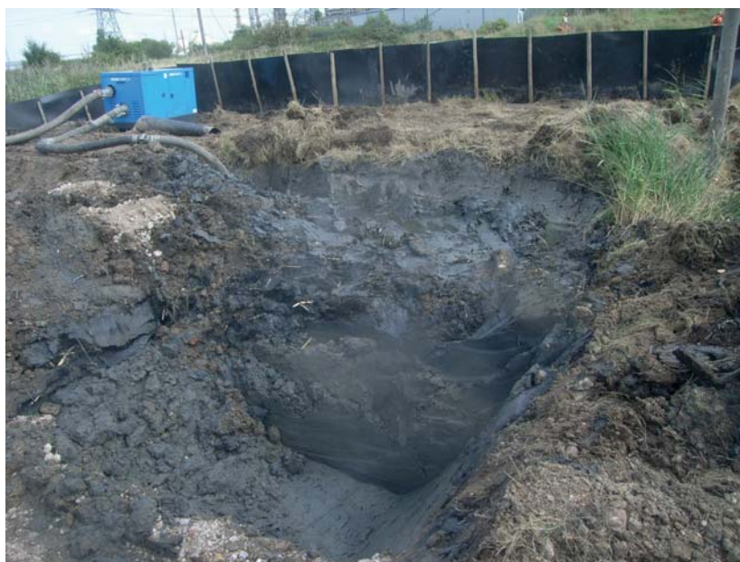
Plate 1: Cable trench excavation in progress, showing undisturbed alluvium close to present ground surface
