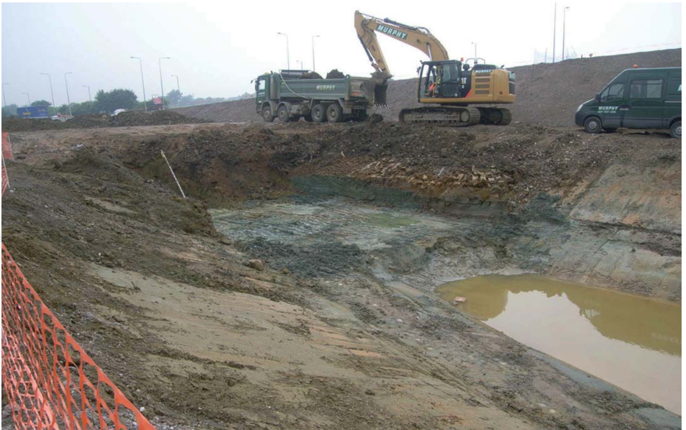
Plate 1: Drainage pond under excavation, general view SW
