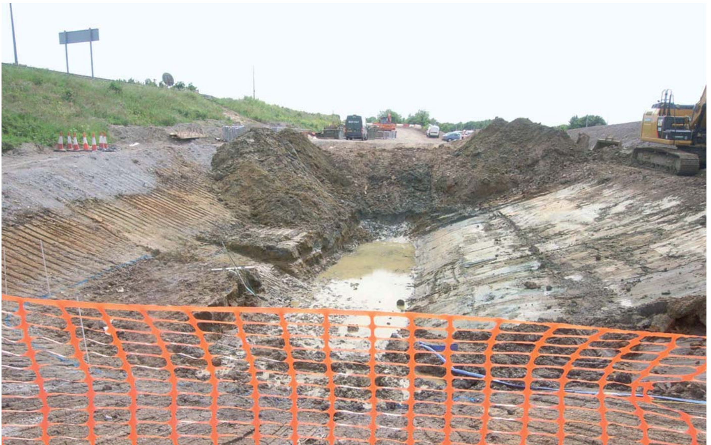
Plate 2: Drainage pond under excavation, general view NE
