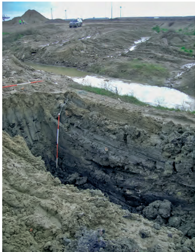
Figure 2.17 A trench exposing thick alluvial deposits during the evaluation at the Logistics Park Infrastructure site
