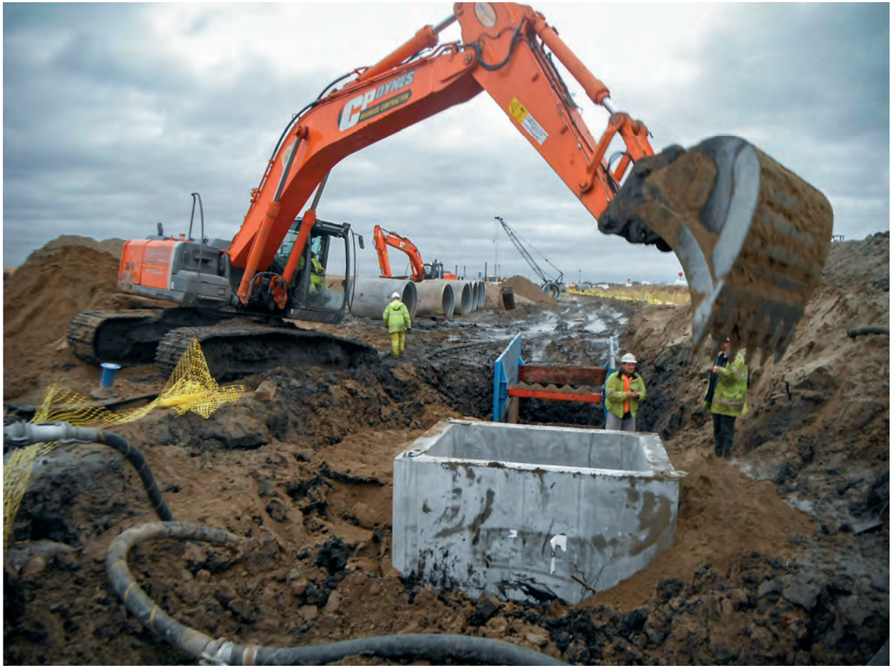
Figure 2.13 Monitoring deep drainage excavations at DP World London Gateway Port Gate Complex
