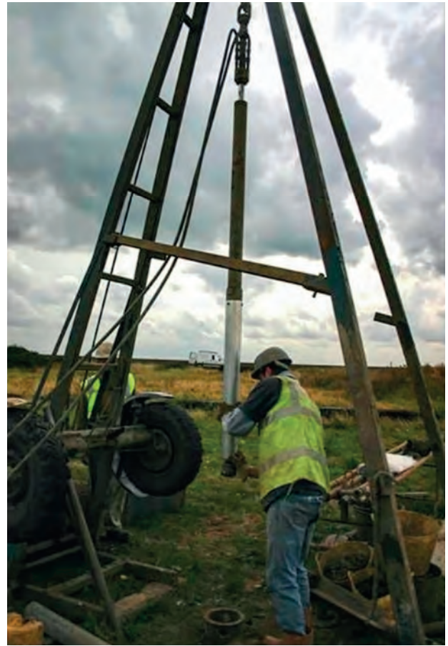
Figure 2.4 The shell-and-auger drill rig in operation
