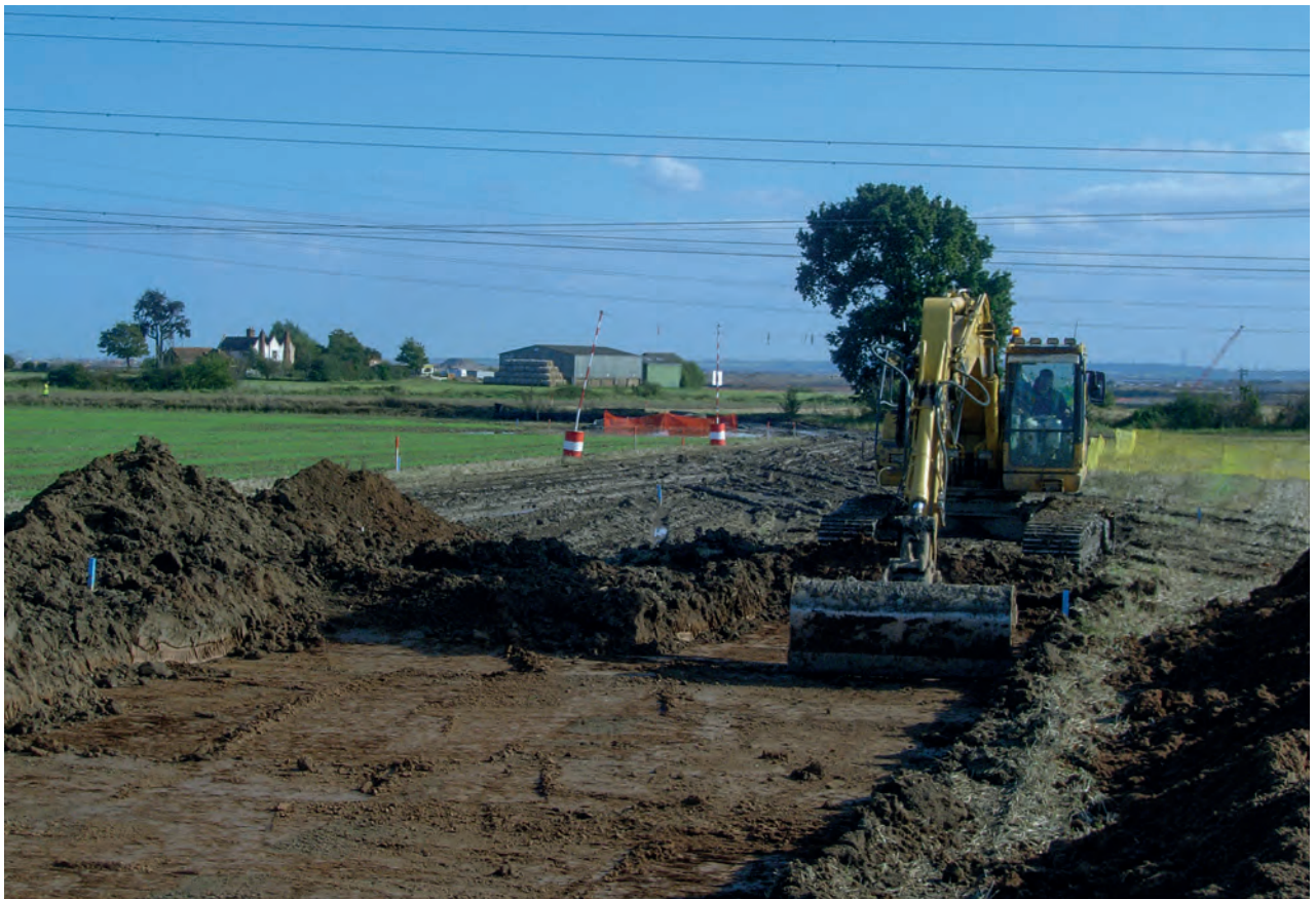
Figure 2.10 Removing the topsoil across Area A on the Access Road
