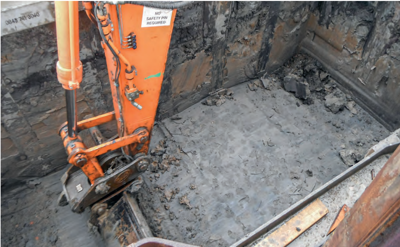
Figure 2.11 Separator pit under excavation, Welfare and Workshop Building drainage
