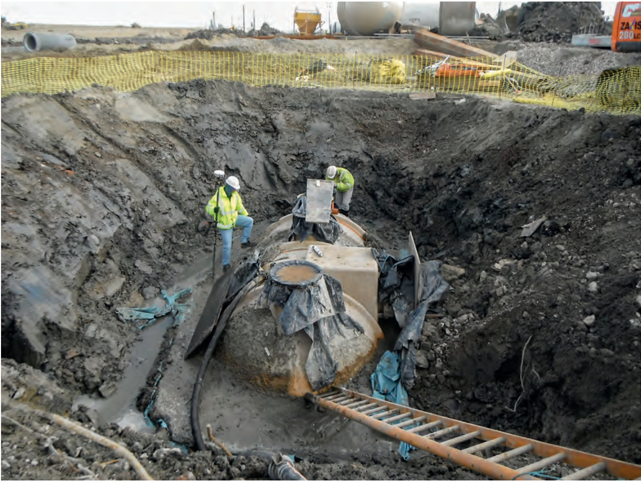
Figure 2.14 Deep drainage excavations in progress at DP World London Gateway Port Gate Complex
