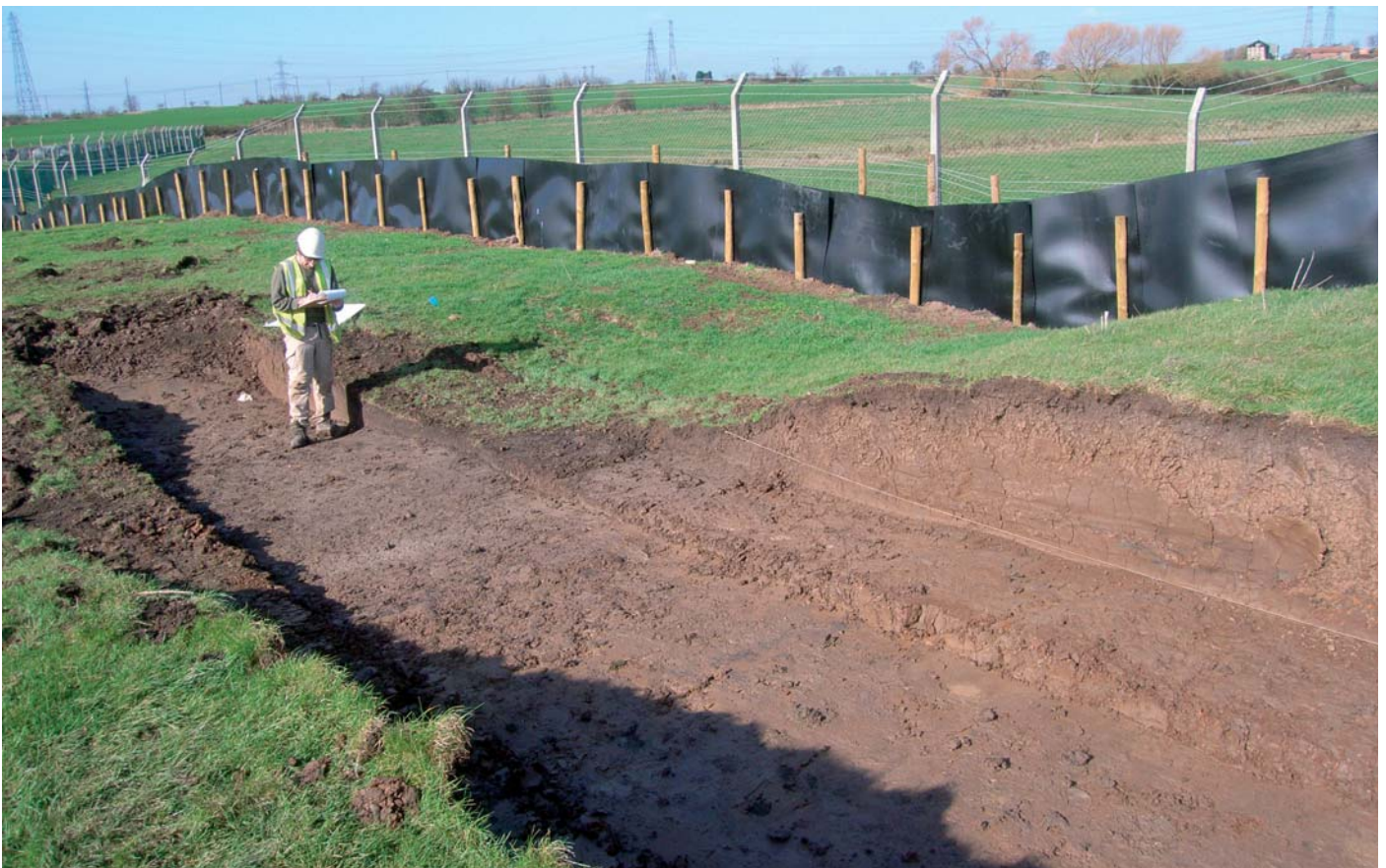
Plate 2: Phase 1 mitigation, historic sea wall section
