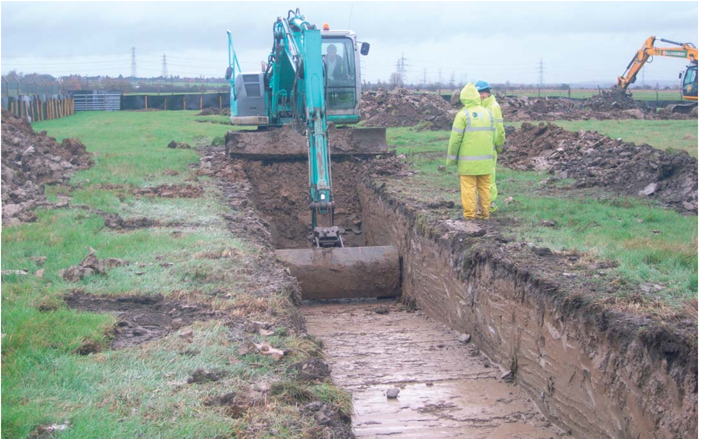
Plate 1: Phase 1 mitigation trenches under excavation
