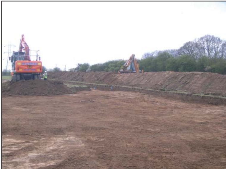
Plate 7: General view illustrating soil stripping conditions Area 1
