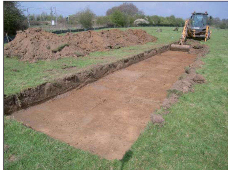
Plate 8: General view illustrating soil stripping conditions Area 2
