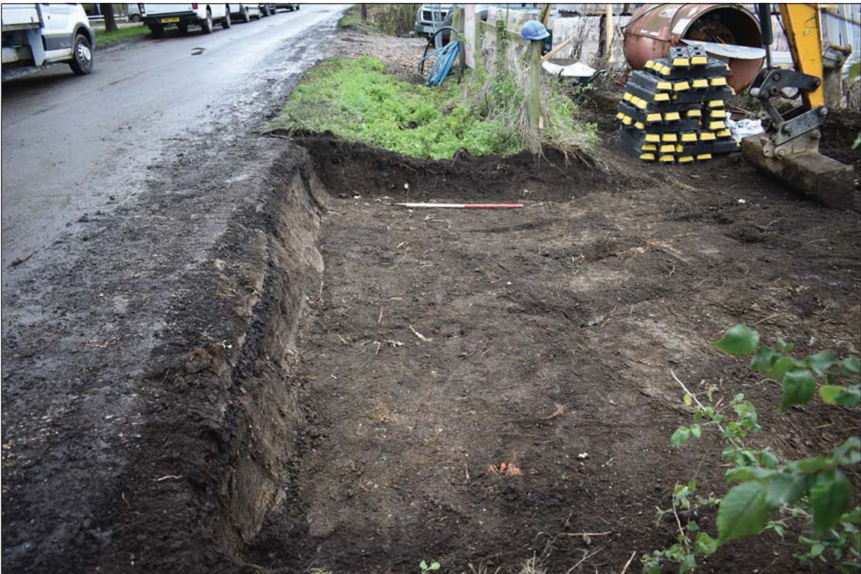
Plate 2: Southern edge of Trench 1, showing the cut for the road (962) and the extant ditch (964), looking south
