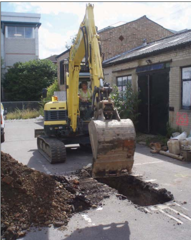
Plate 2: Excavation of test pit 4
