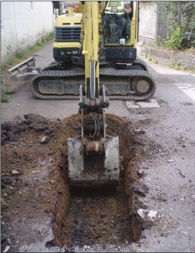
Plate 1: Excavation of test pit 2
