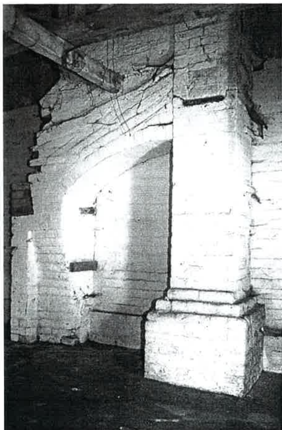
Plate 17: Chimney stack within lean-to to rear of Kiln 2
