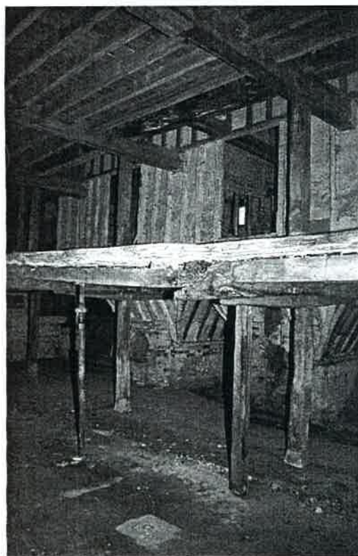
Plate 7: View towards Kilns 3 and 4 from within area of collapsed first floor
