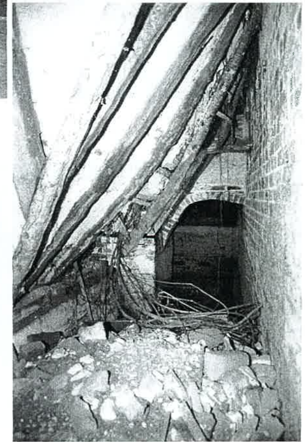
Plate 12: Curved flue to rear of Kiln 2
