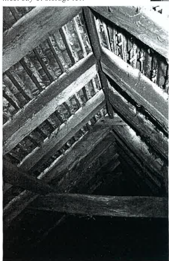
Plate 15: Ridge-piece within northernmost bay of storage loft
