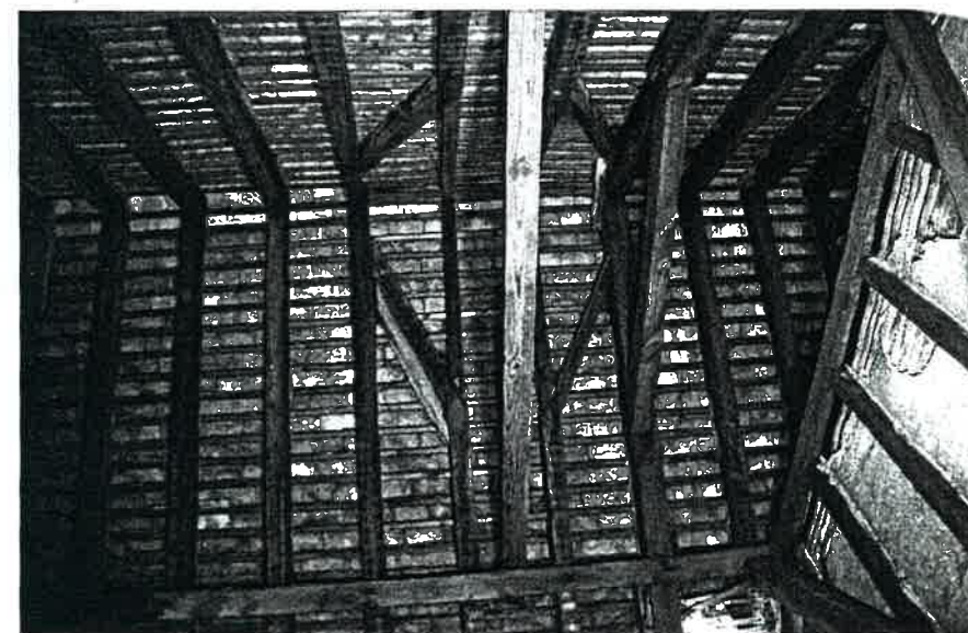
Plate 8: Angled supports between rafters for former cowlf above Kiln 2
