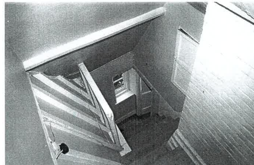
Plate 14: View down cottage stairs from second floor
