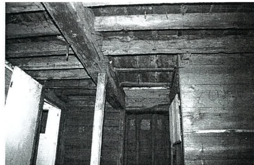
Plate 16: Section of floor structure within F3 without floor joists
